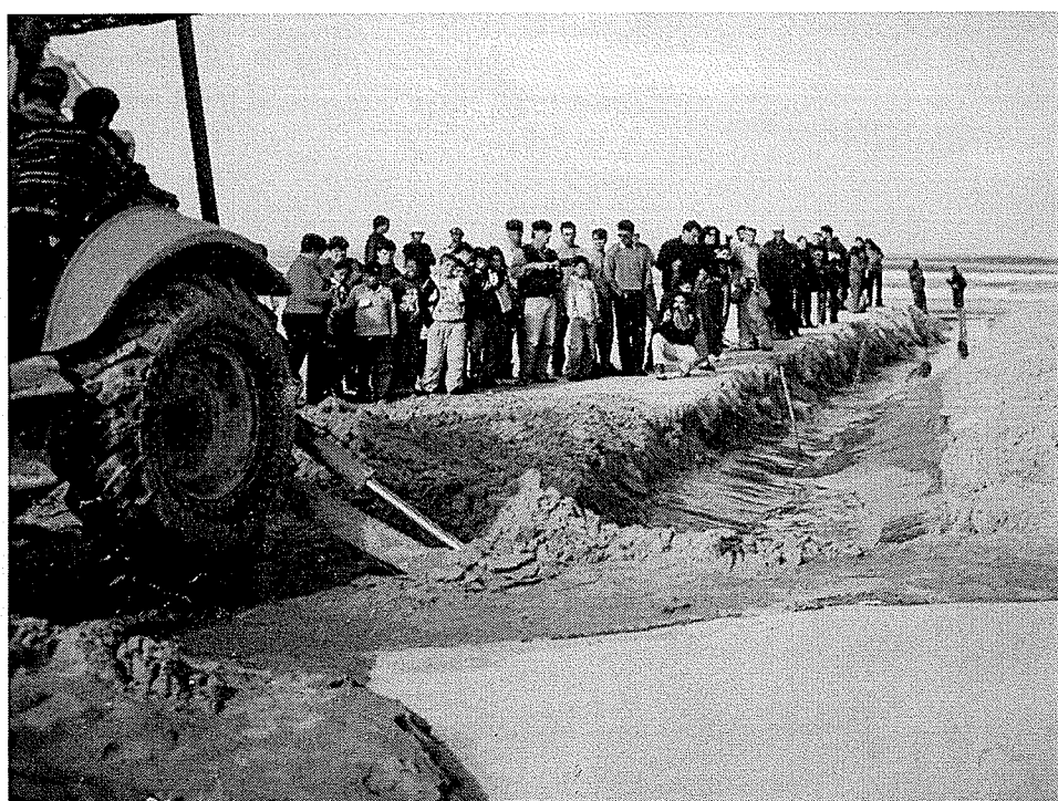
Figure 13: Backhoe opening the Lagoon mouth
