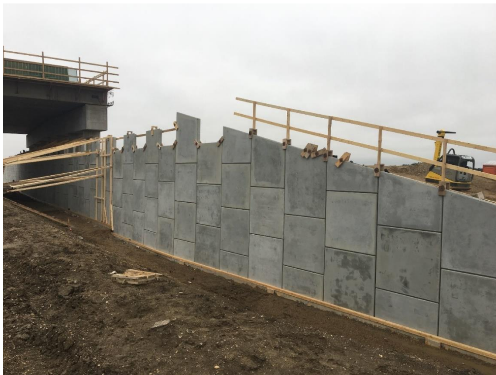
Figure A-10 – South Wall Construction Progress as of June 2, 2018
