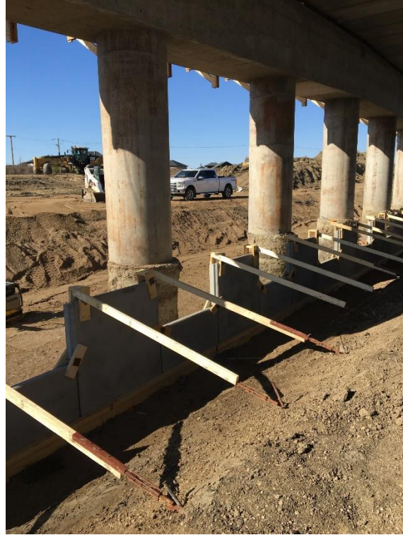
Figure A-7 – Front Facing of North Abutment Wall Panels (Centre Section)
