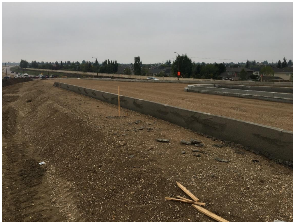
Figure A-20 – North Embankment Construction Progress as of August 28, 2018
