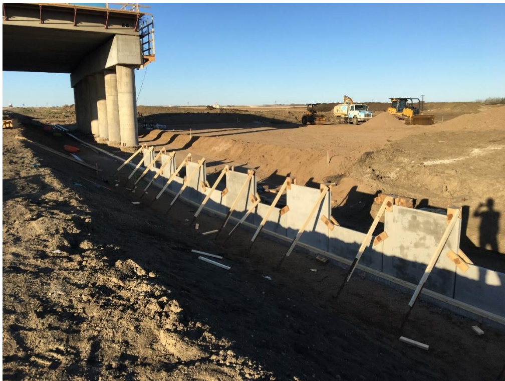
Figure A-6 – Front Facing of South Abutment Wall Panels
