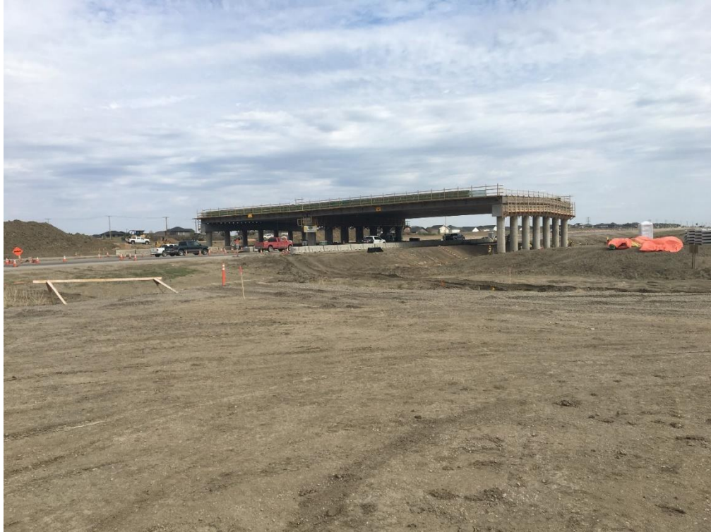
Figure A-1 – Bridge Interchange Site as of May 9, 2018
