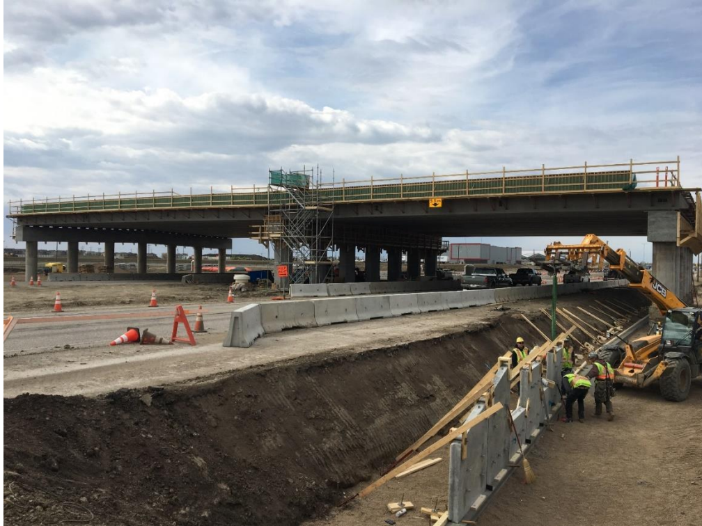
Figure A-5 – Process of Wall Panel Placement
