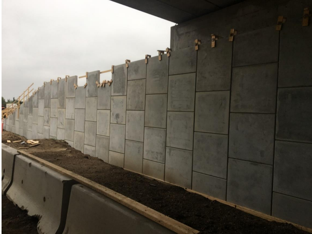
Figure A-11 – North Wall Construction Progress as of June 2, 2018
