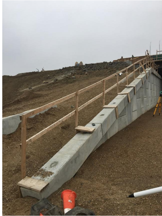
Figure A-19 – North Embankment Elevation as of August 28, 2018
