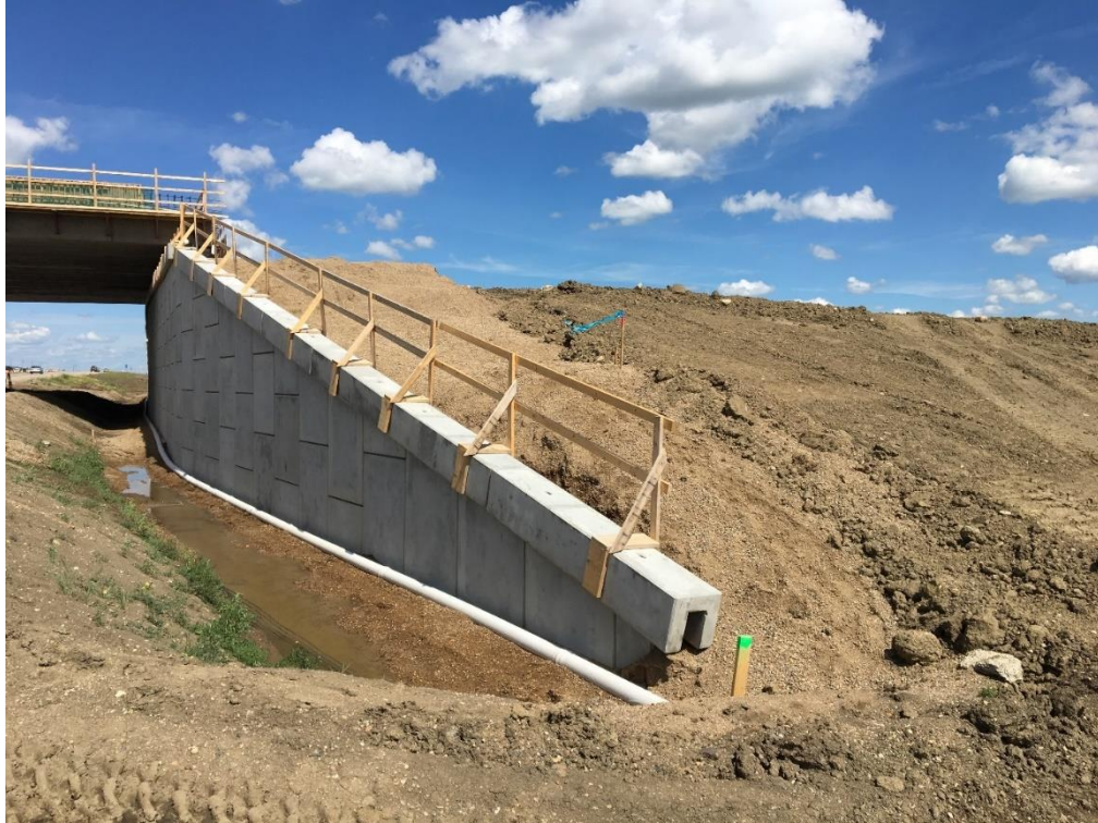
Figure A-15 – Profile View of South Abutment as of July 5, 2018
