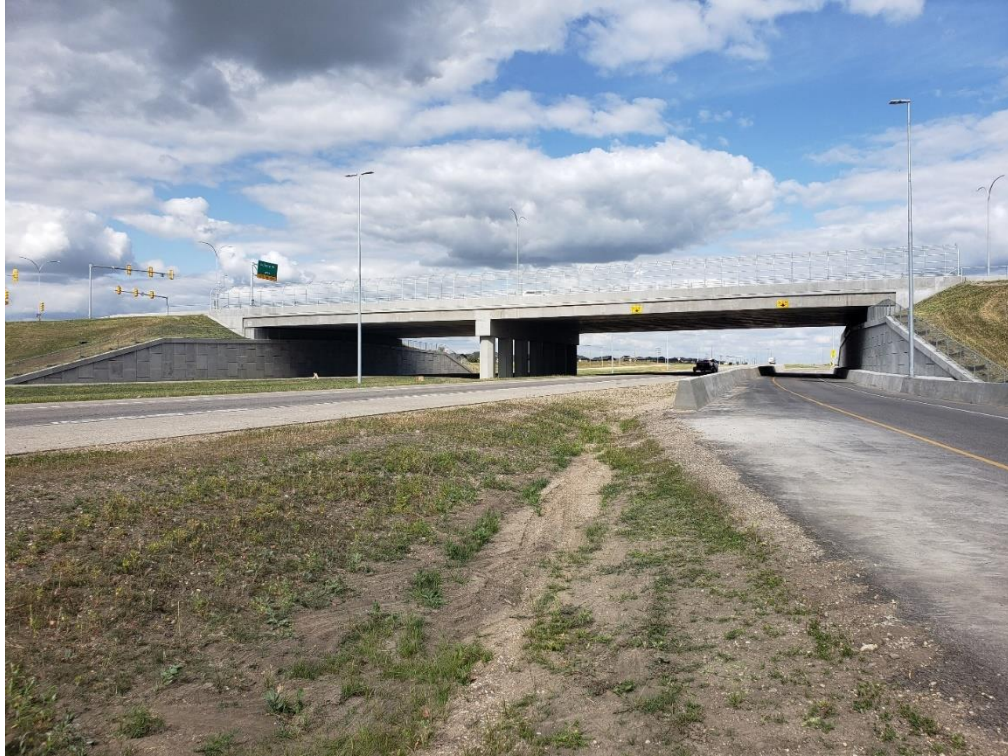
Figure A-21 – Completed Bridge Interchange as of August 13, 2019
