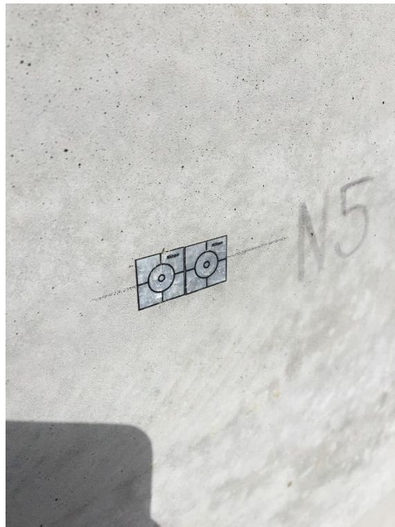
Figure A-16 – Survey Targets for Wall Measurements
