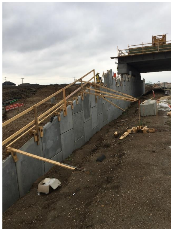
Figure A-8 – North Wall Construction Progress as of May 25, 2018
