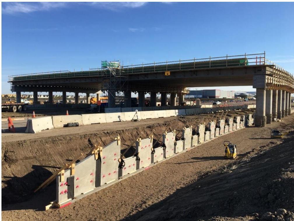
Figure A-4 – Back-Facing of North Abutment Wall Panels
