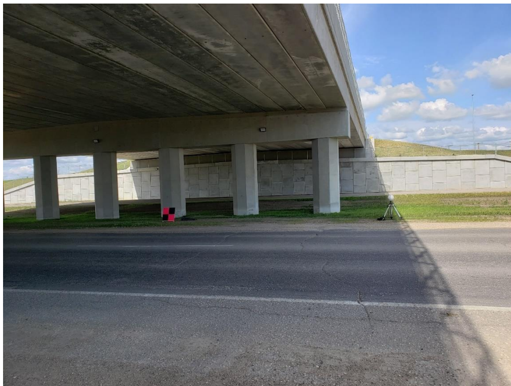
Figure A-23 – Middle Pier View Facing South Abutment as of August 13, 2019
