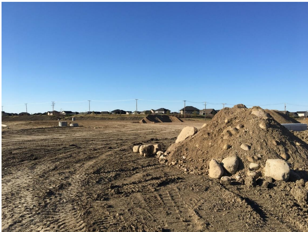
Figure A-2 – North Approach Embankment Progress as of May 9, 2018
