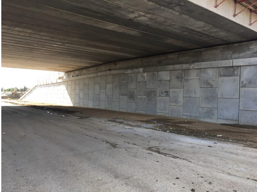
Figure A-17 – North Wall Construction Progress as of August 28, 2018
