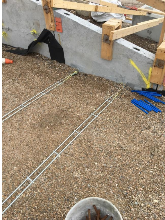
Figure A-9 – Metallic Strip Reinforcement
