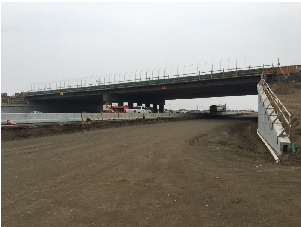
Figure A-18 – Bridge Interchange Construction Progress as of August 28, 2018
