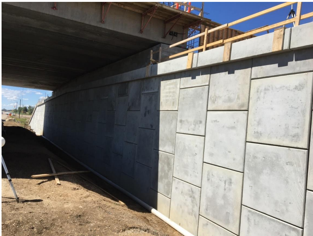
Figure A-14 – North Wall Construction Progress as of July 5, 2018
