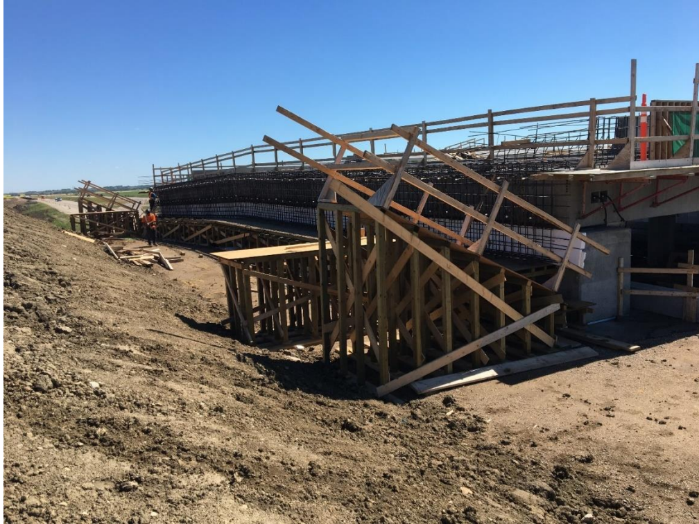
Figure A-13 – Construction of Embankment/Bridge Deck Construction on July 5, 2018
