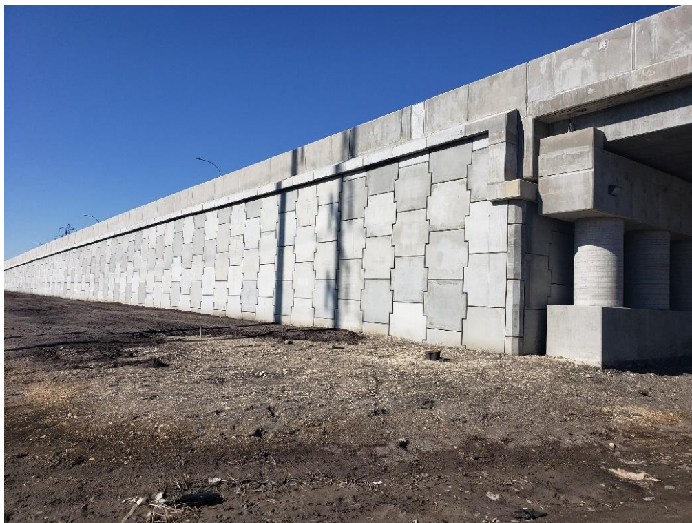
Figure 2-1 – Mechanically-Stabilized Earth Retaining Wall Structure
