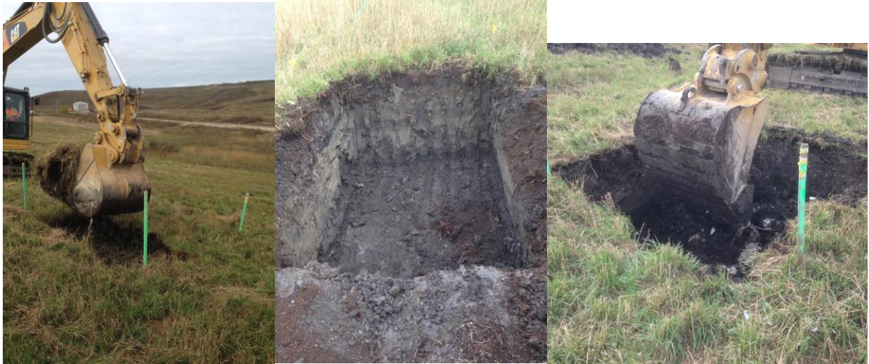
Figure A -1. From left to right, digging the hole, the hole with 1.3 m depth, filling the bio-window with compost
