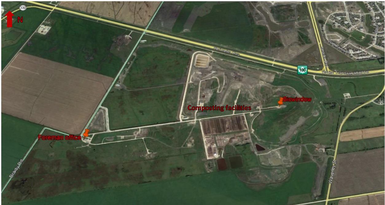
Figure C- 1. The BRRMF with composting windrows and the location of the biowindow (Google, n.d.)
