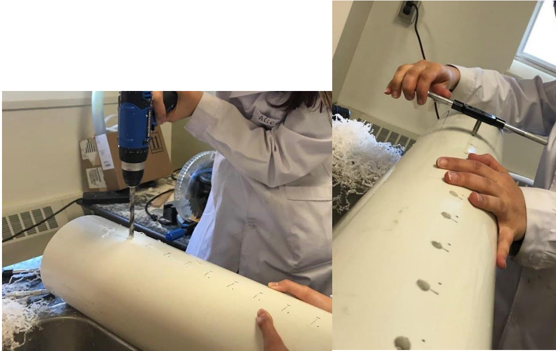
Figure B- 11. Drilling and threading the holes in the PVC pipe for installation of gas sampling ports
