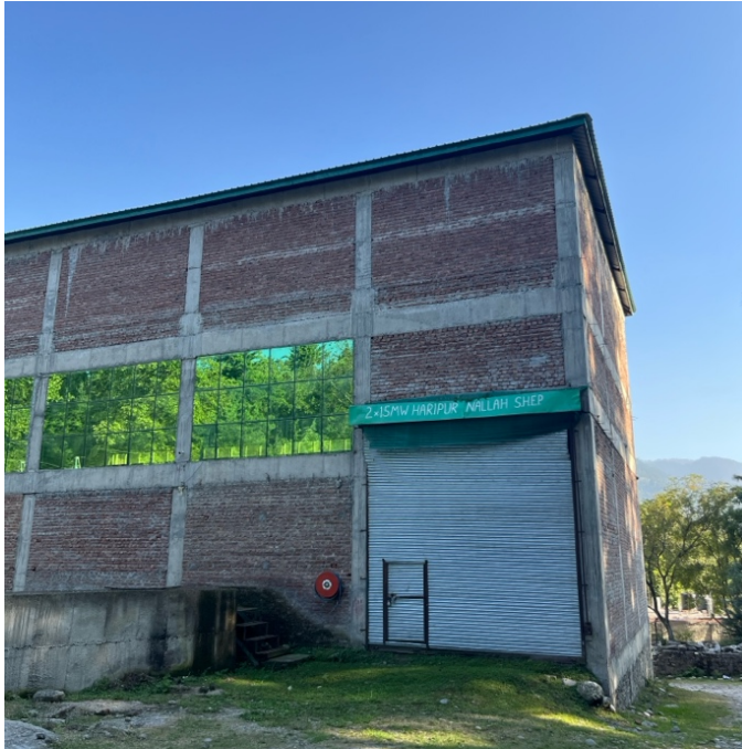
Haripur Nallah Project Amongst a Forested Area
