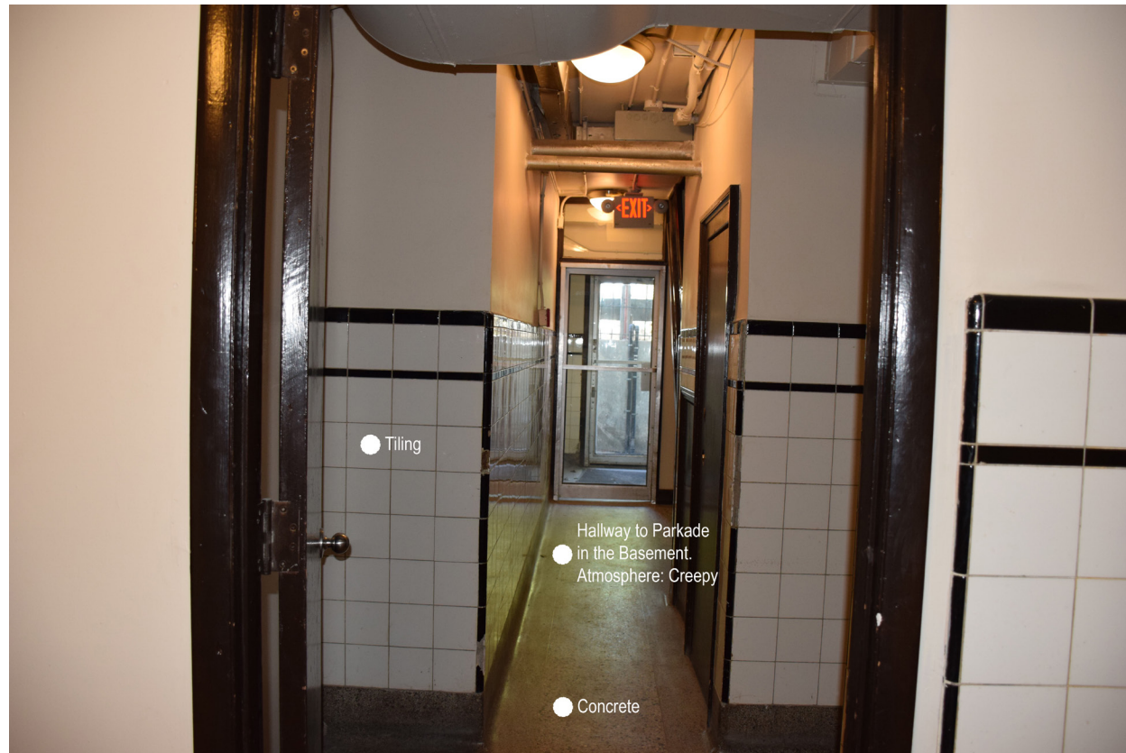
Figure 52: Photograph showing the Exit from the Basement into the Parkade.
