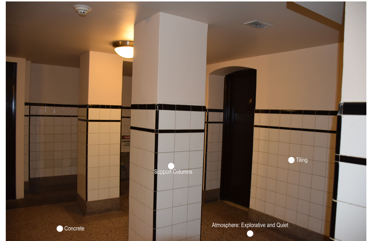
Figure 53: Photograph showing the Hallway in the Basement.
