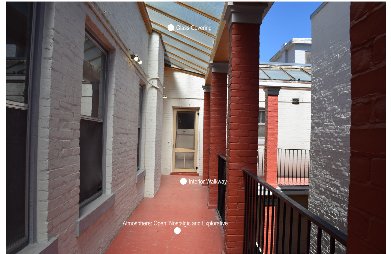
Figure 57: Photograph showing the Interior Walkway Facing the Interior Courtyard.
