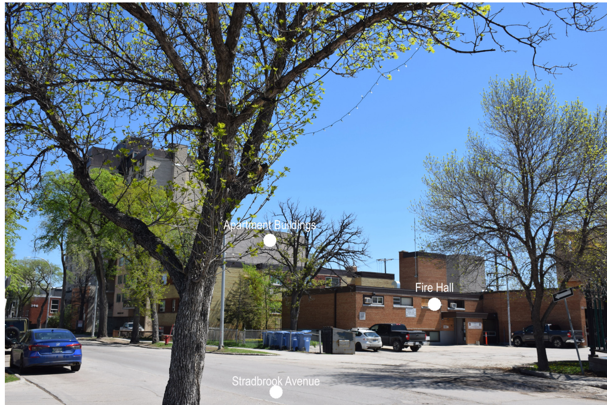
Figure 49: Photograph showing the Entrance into the Route along Stradbrook Avenue after Stradbrook at Osborne.
