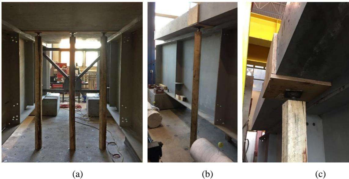
Figure 3.26 Deck joint formwork.
