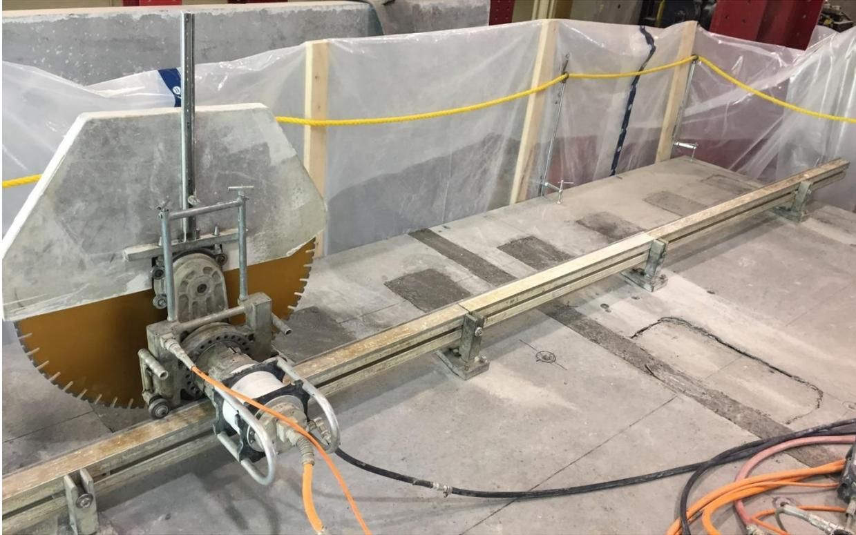
Figure 4.35 JPD demolition setup with concrete water saw.
