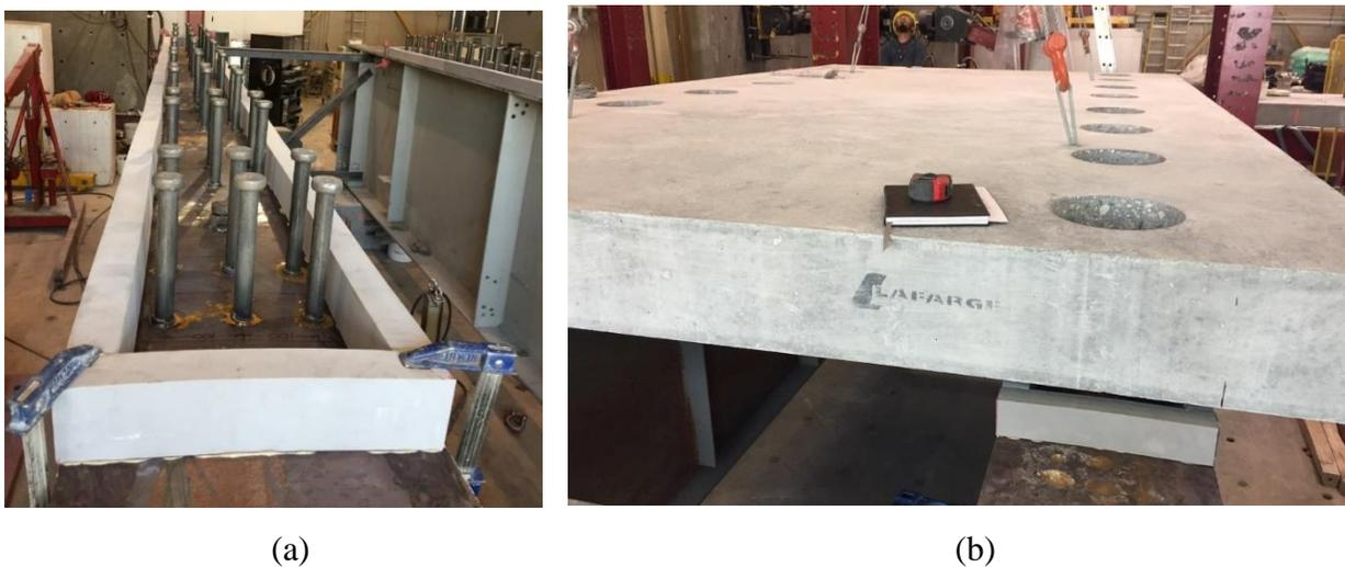
Figure 3.28 The bridge deck haunch construction: (a) EVA foam installation; (b) placing FPD.
