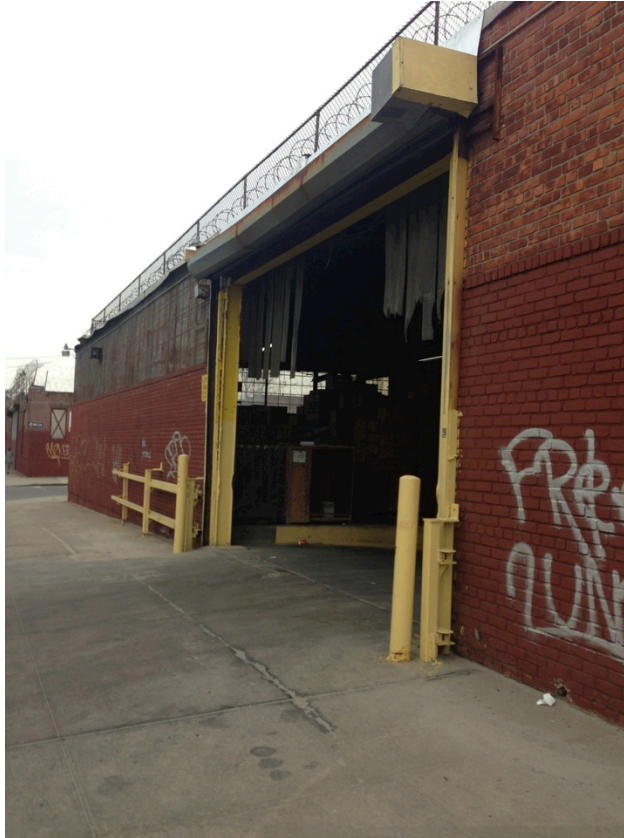
Figure 31. Interior Loading Dock on McKibbon Street.
