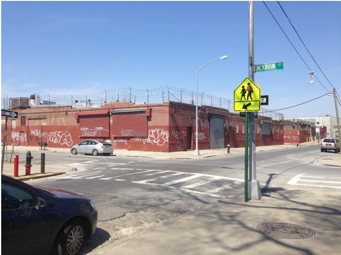
Figure 30. Corner view of 71 White Street at McKibbin Street.
