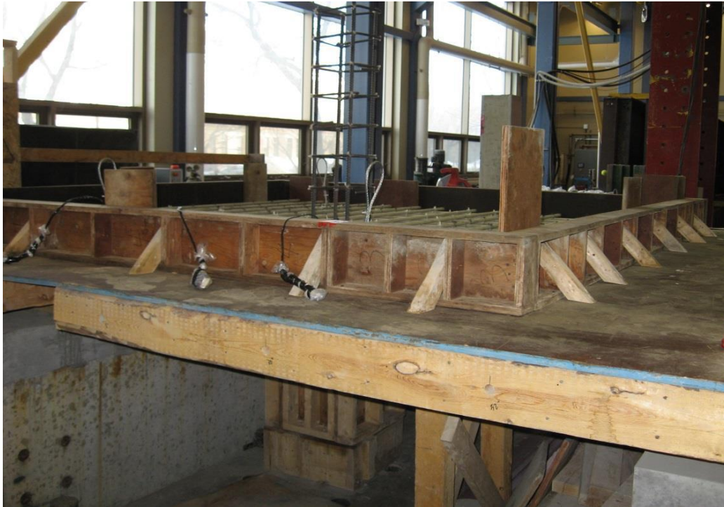
a) Photo for the formwork
