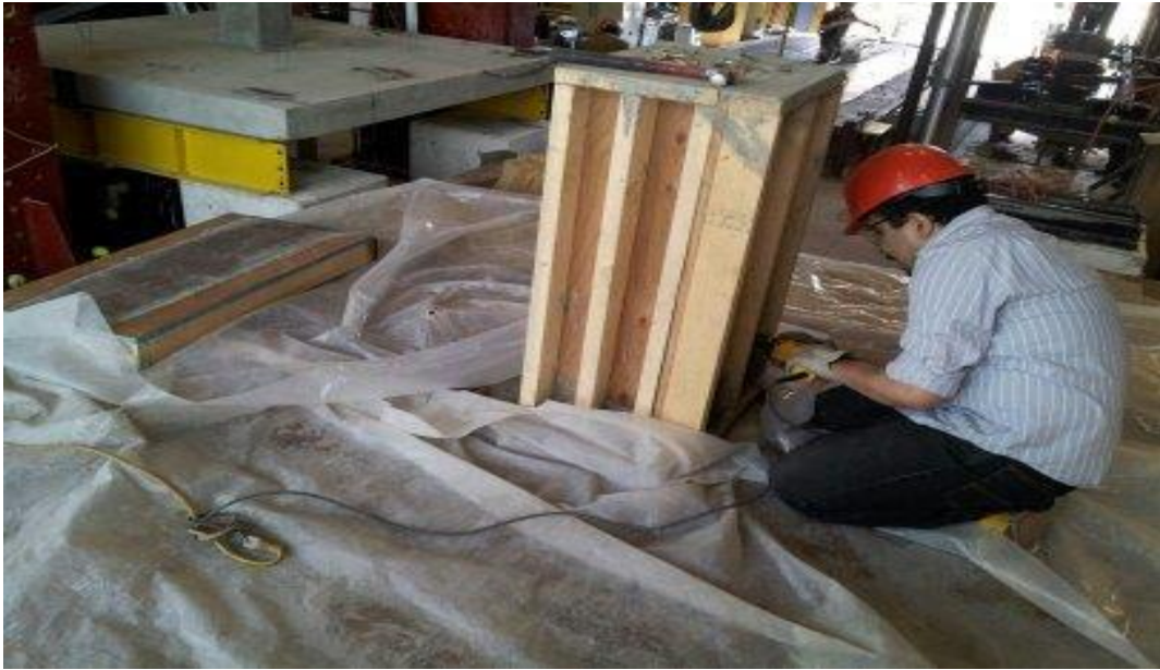
Figure 3.11: Curing of the slabs
