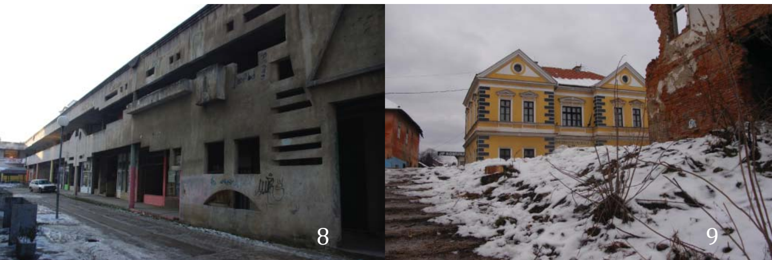
8. Partially completed two level 'strip mall' some interior spaces are completed and occupied, others are concrete shells.
