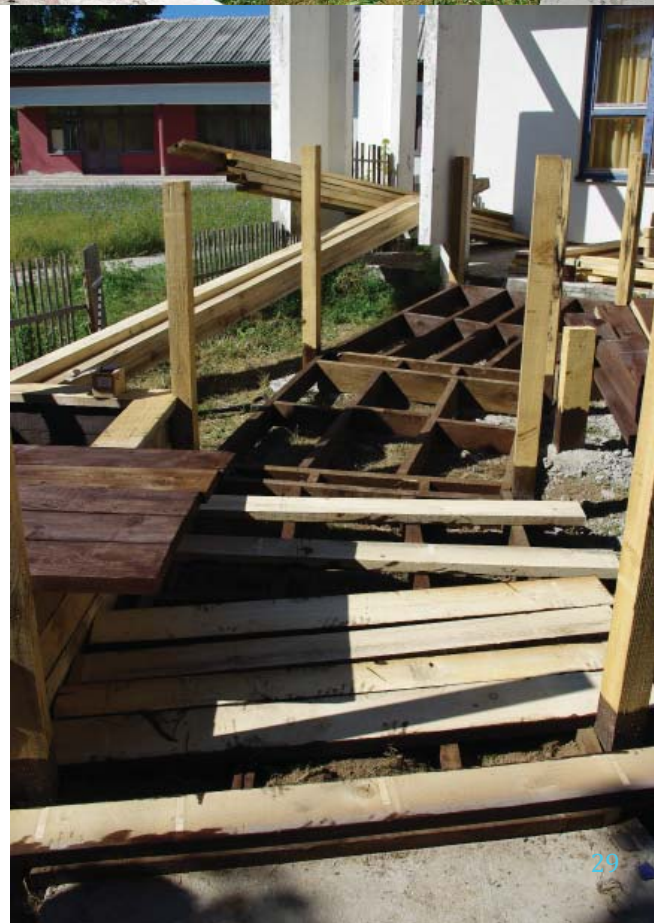
Figure 1.15 Construction of the curving ramp.
