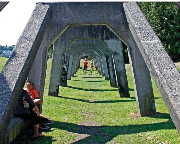
Figure 2.13** Concrete Tressle, Gasworks Park, Seattle.
