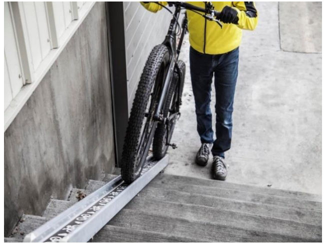
Fig. 122 Rail fastened to the stair / Access to the Baana, Helsinki
