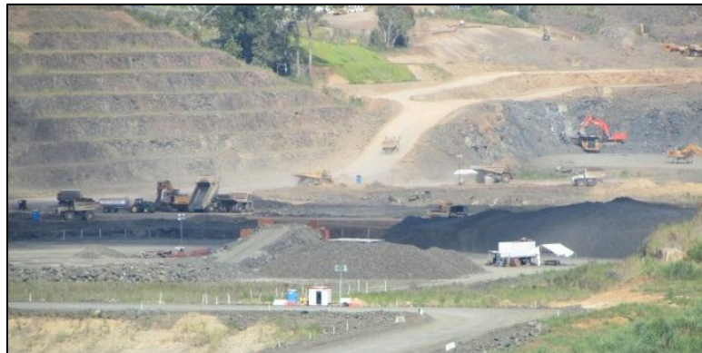
Figure 34: Panama Canal Expansion Progress
