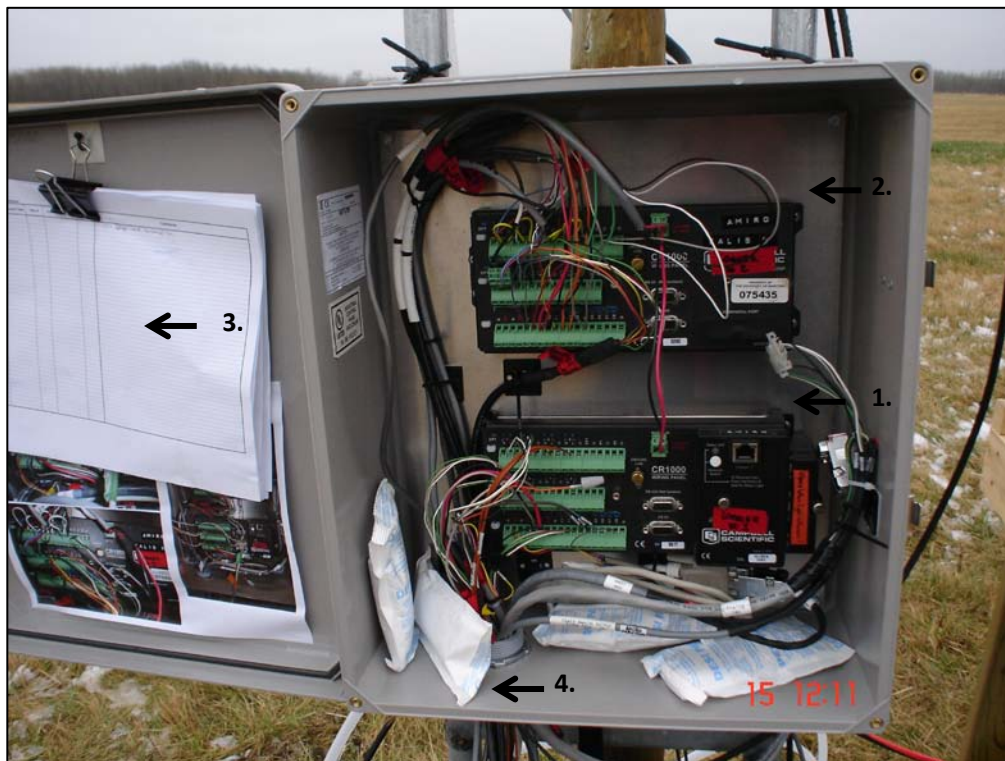
Figure A 3. The Treatment Field Logger Box.
