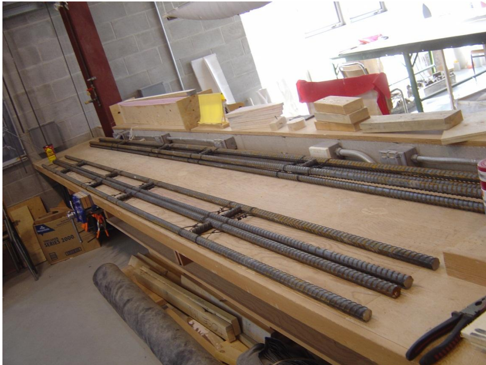
Figure 4.22 – Reinforcement preparation, 2-25M bars
