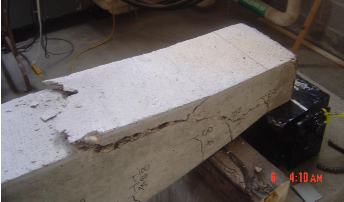
Figure 5.27 – Failure close-up for CB1
