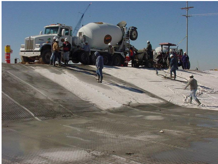
Figure 3.2 – Unimat Revetment reservoir lining, both before and after concrete pour (Fabriform)
