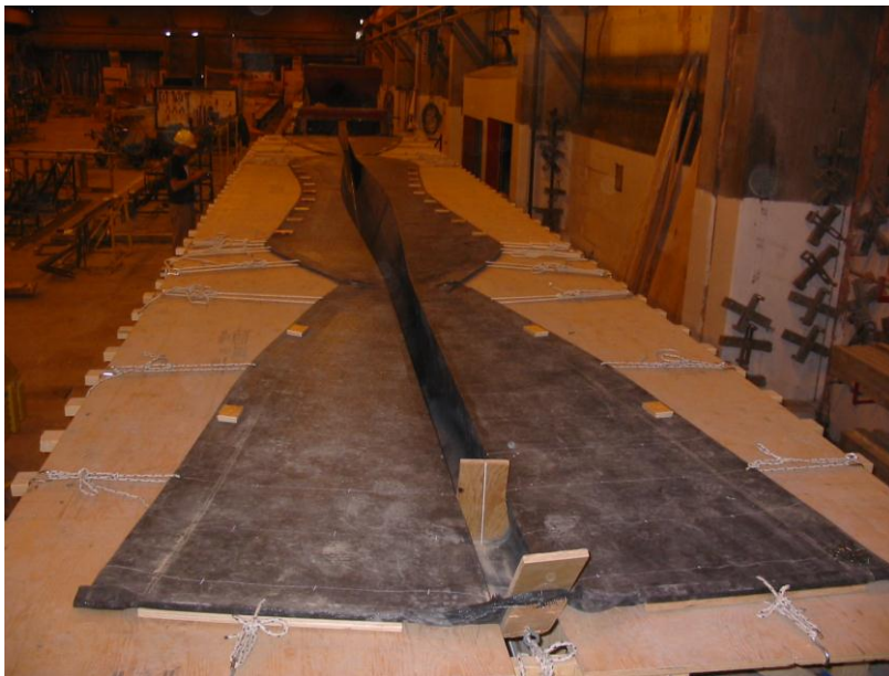
Figure 3.14 – Formwork for the fabric formed concrete beam
