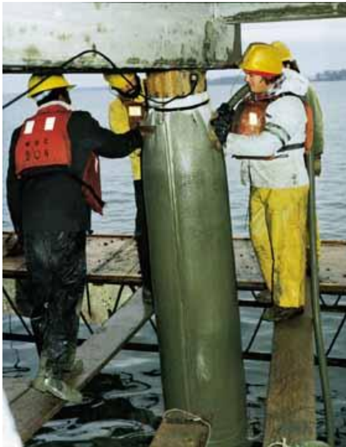
Figure 3.5 – Installation of pile jacket, (Fabriform)
