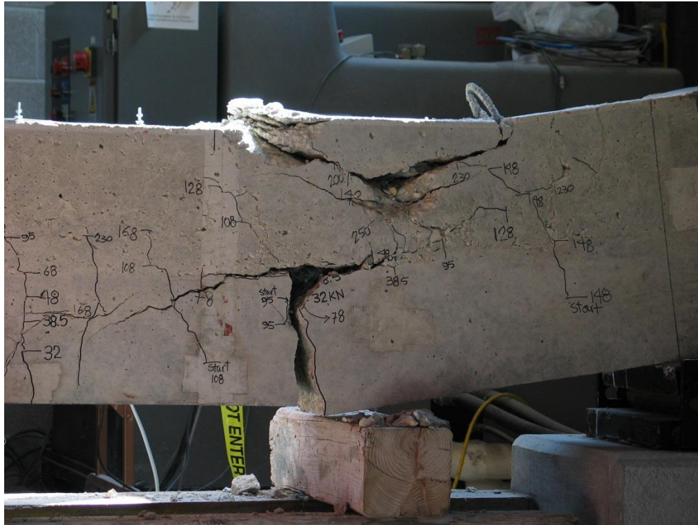
Figure 5.63 – Close-up of failure
