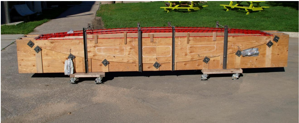
Figure 4.50 – Modified formwork to fabricate CCB's
