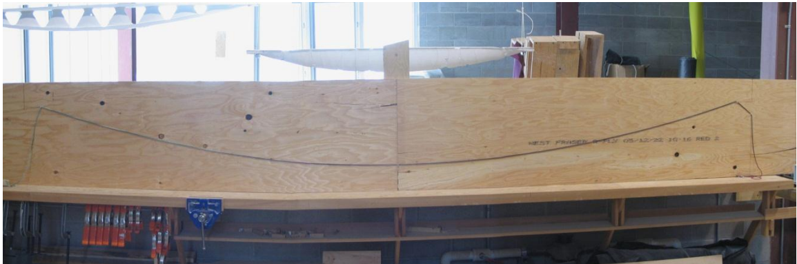
Figure 4.4 – Catenary curve for the construction of formwork
