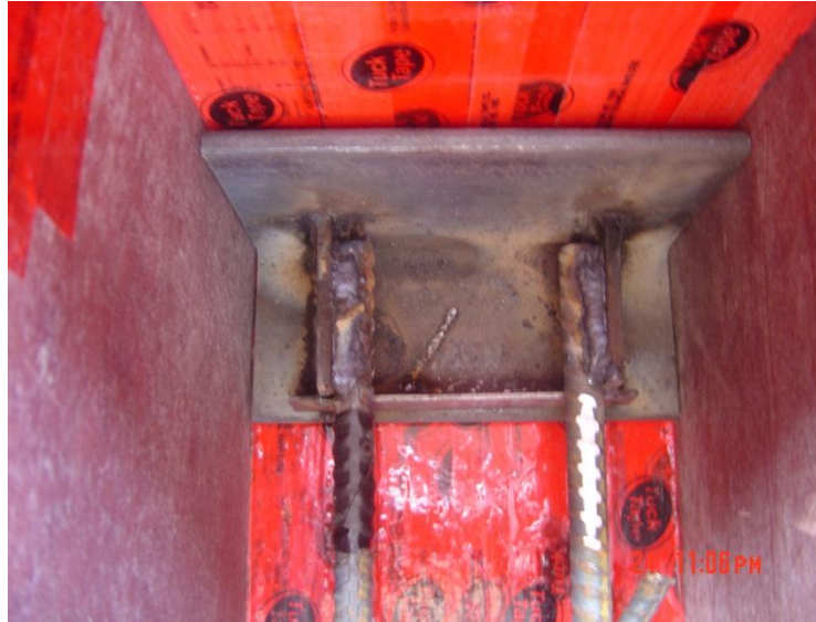
Figure 4.34 – End-angle detail for RB4
