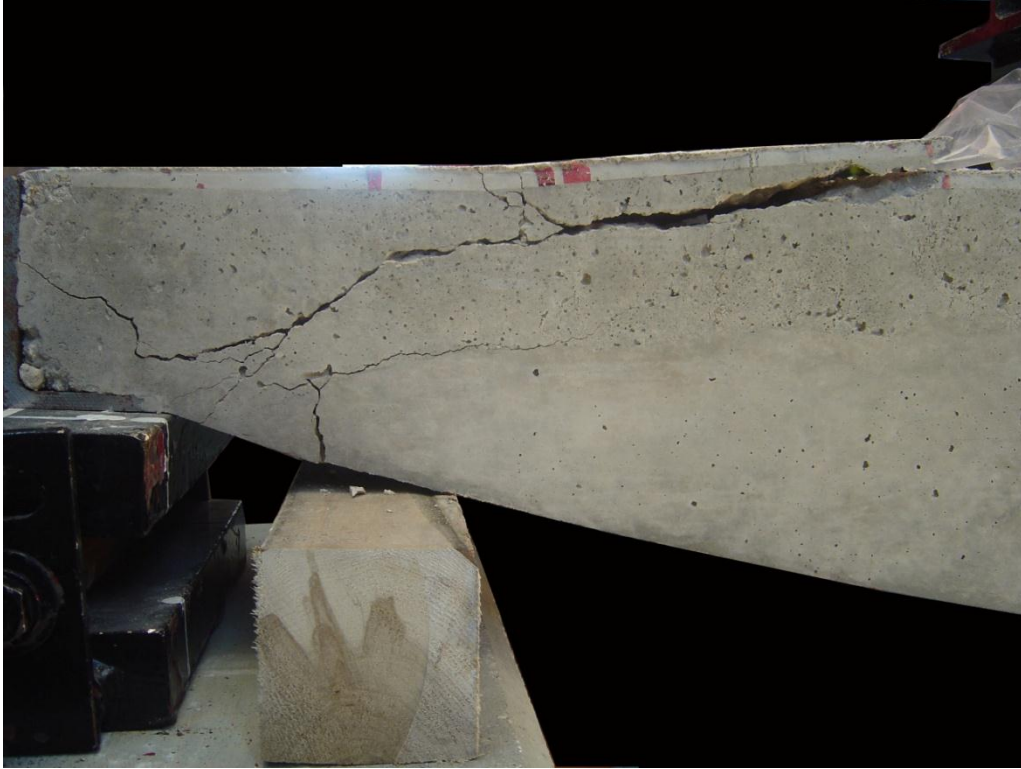
Figure 5.21 – CB1's end failure
