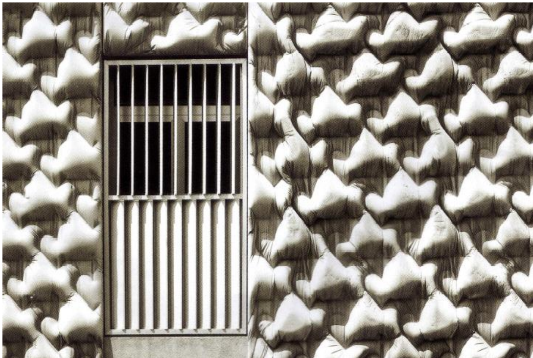
Figure 3.8 – Wall panels after construction, Hermanas Hospitalarias Social Centre project, Madrid 1985 – 1986, by M. Fisac (AV 2003)
