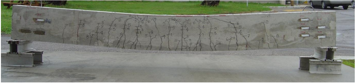
Figure 5.80 – RB4 after failure
