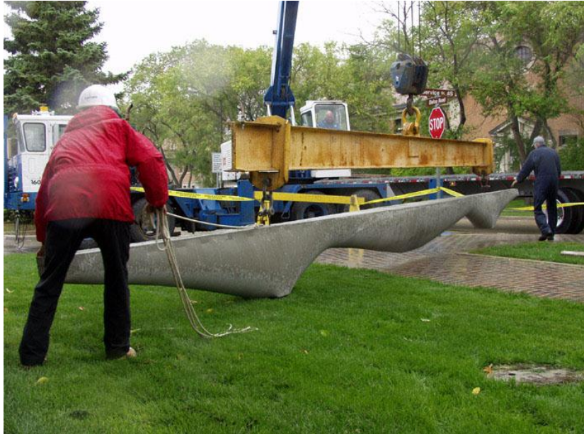
Figure 3.13 – Fabric formed concrete beam
