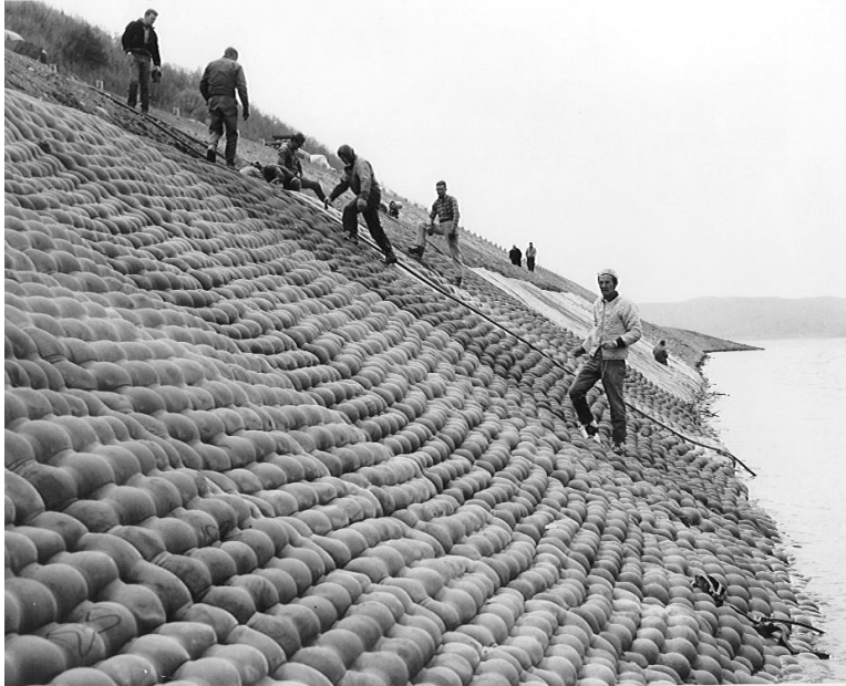
Figure 3.1 – Filterpoint soil erosion prevention, installed in 1967 on the Allegheny Reservoir New York (Fabriform)
