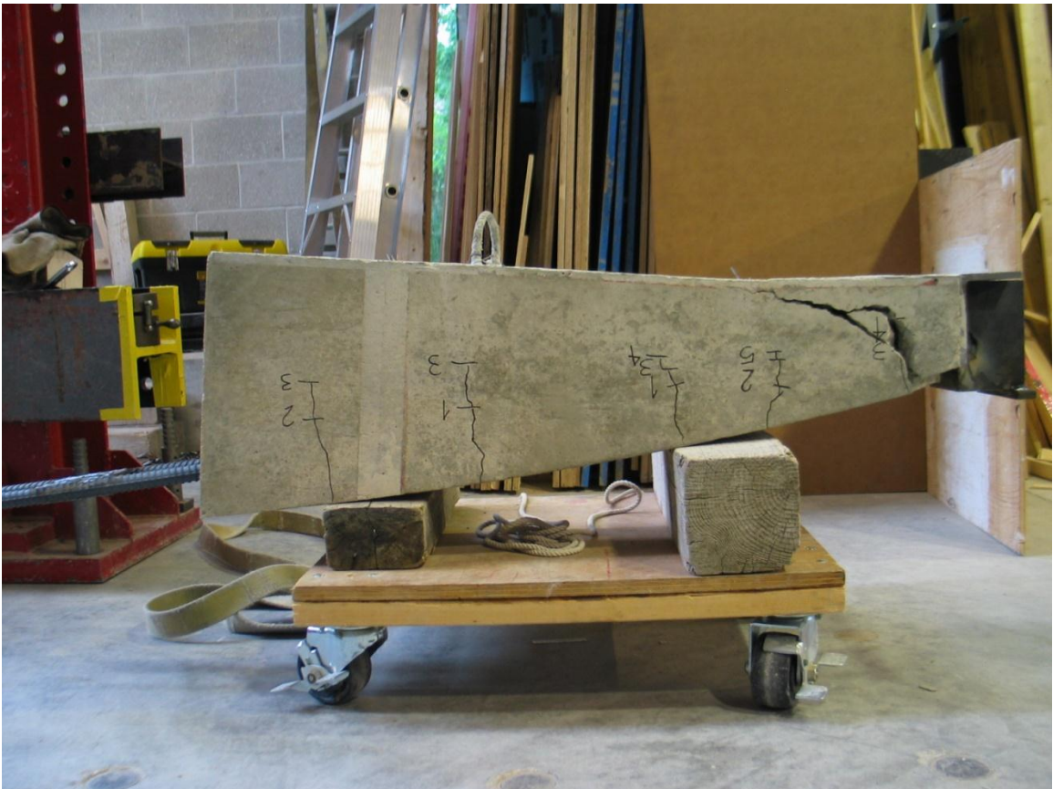
Figure 5.99 – ECB-TS-RA1 after testing
