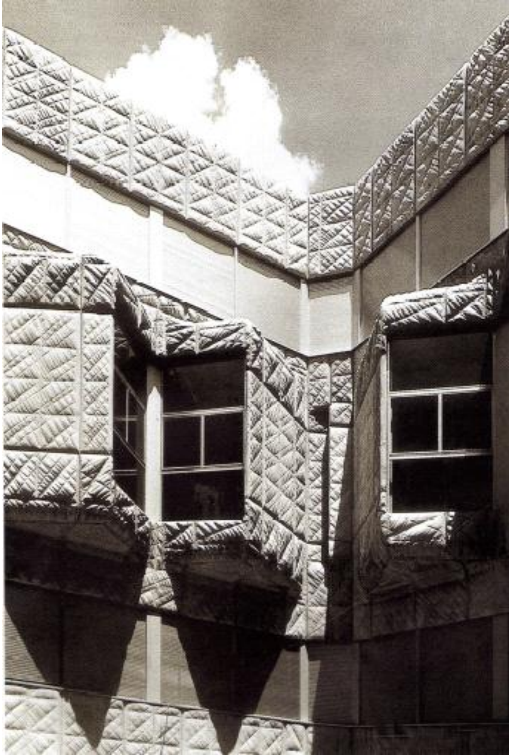
Figure 3.6 – Mupag Rehabilitation Centre, Madrid 1969 – 1973, Architectural wall panels by M. Fisac (AV 2003)
