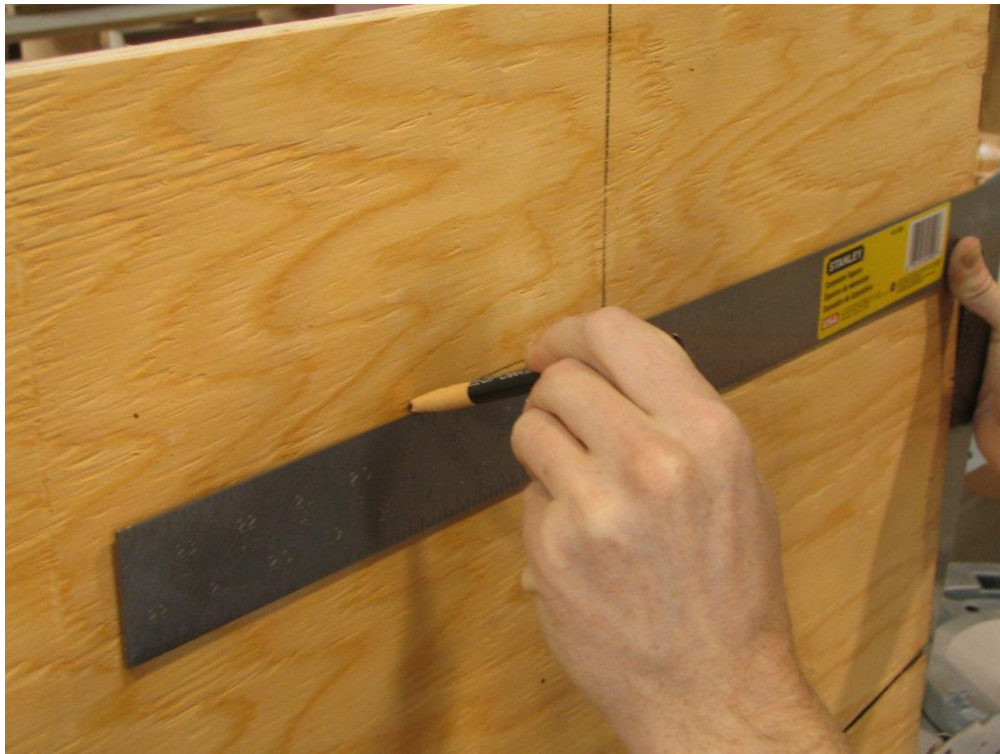
Figure 4.5 – Drawing the beam profile on the side wall of the formwork (scale 1:1)
