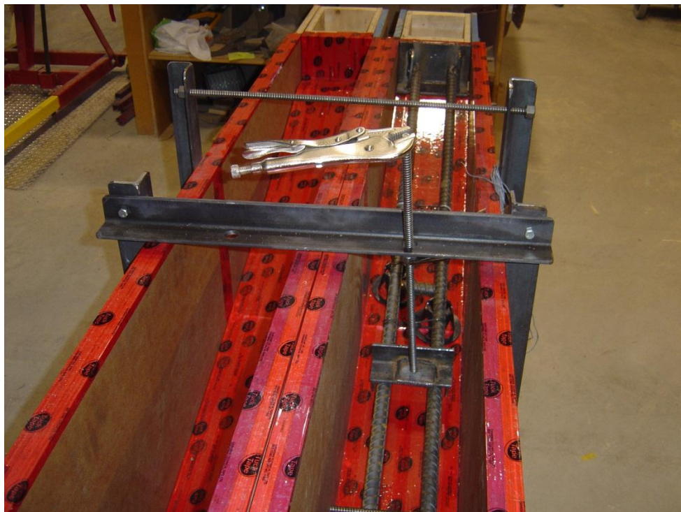
Figure 4.24 – Reinforcement placement in formwork
