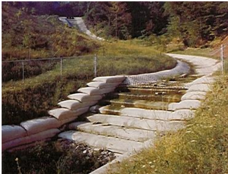
Figure 3.4 – Concrete Bags, (Fabriform)
