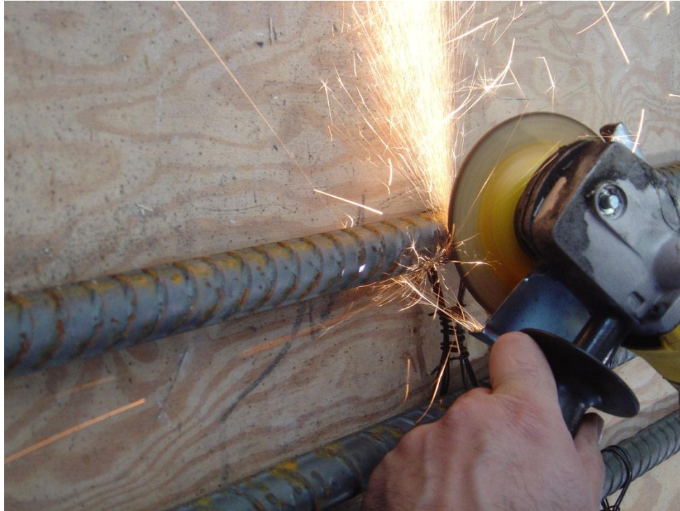
Figure 4.23 – Preparing reinforcement for strain gauge installation
