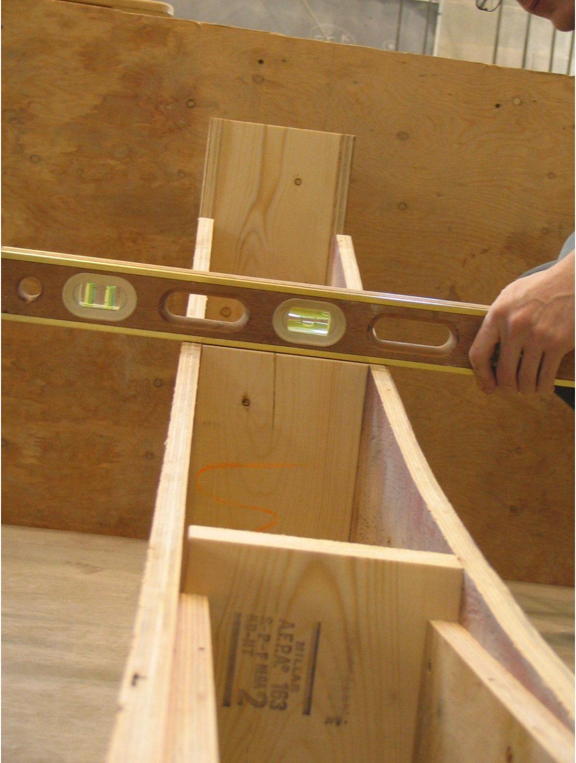
Figure 4.11 – Levelling the sides and quality control
