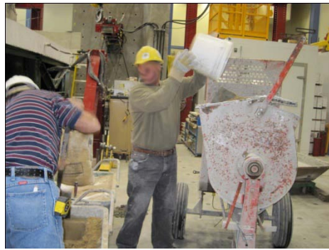
(a) Mixing of mortar
