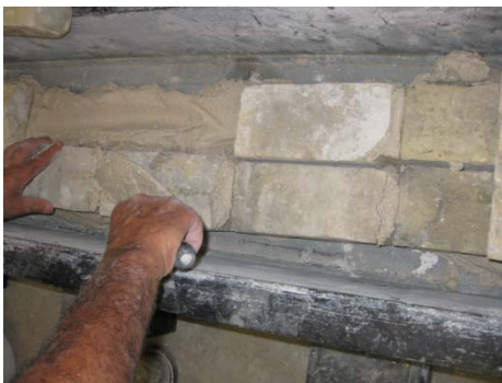
(e) Placing of first brick layer
