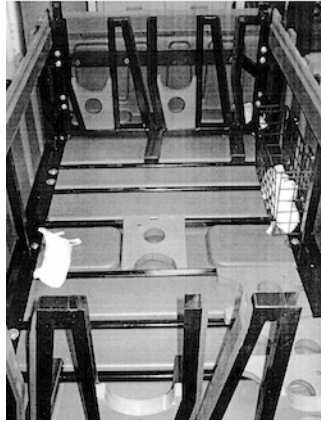
Figure 16: Reinforced metal frame
