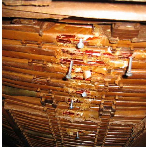
Fig. 4.8: C-phase valve-winding discs exposed to perform pulse injection response tests.
