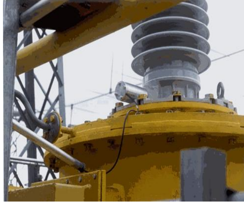
Fig. 4.4: Method of PD coupling through High Frequency Current Transformer terminated on the capacitance-tap of the line-winding transformer bushing
