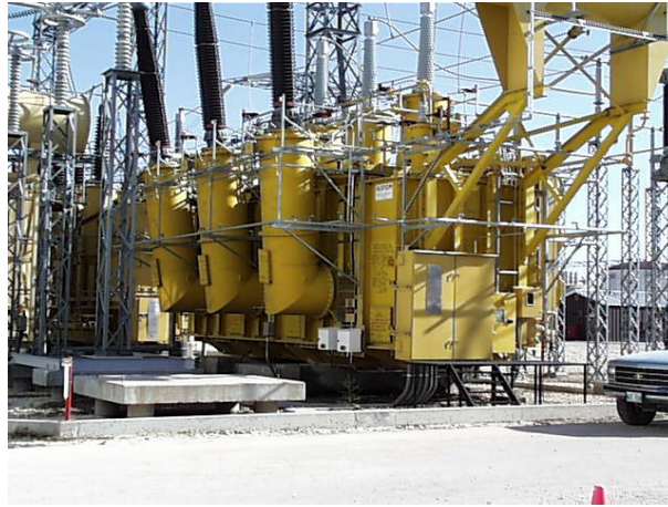
Fig. 4.1: HVDC converter power transformer rated 262MVA, 60Hz, 230kV - 106kV, insulated for 500kVdc. This is a sister unit to the unit which had online PD measurements performed on it and is similar in appearance
