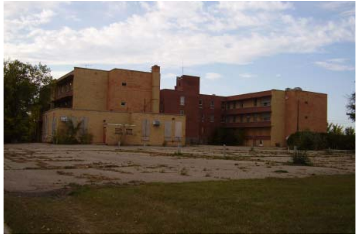
Figure 6 Former St. Peter's Hospital Melville, Saskatchewan Hospital Back East Side
