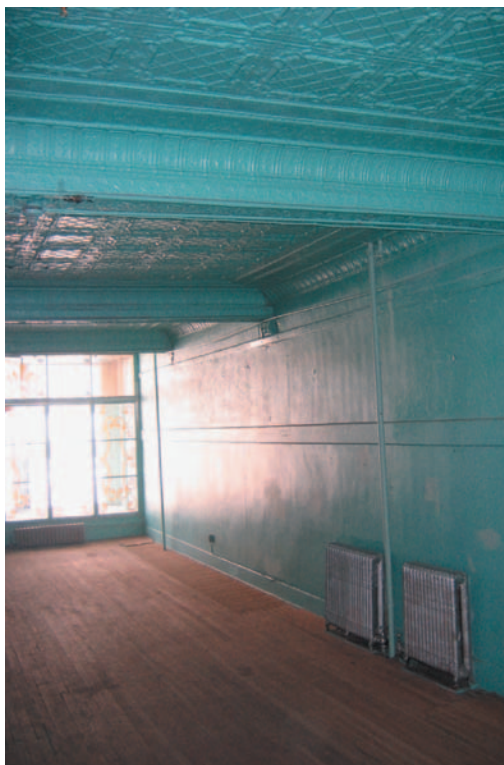
Figure 43: 284 William Avenue: Interior. (Sosa Fontaine, 2010).
