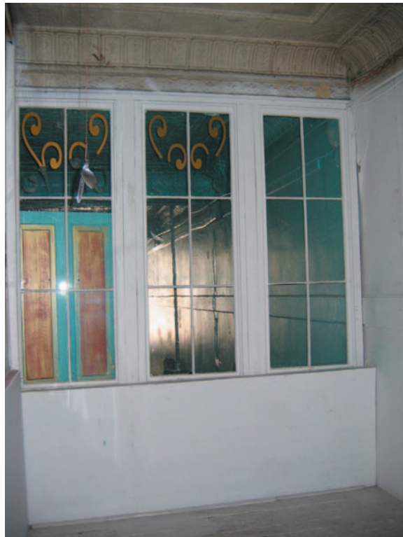
Figure 40: 284 William Avenue: Interior. (Sosa Fontaine, 2010).
