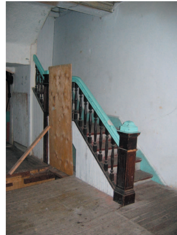
Figure 44: 284 William Avenue: Interior. (Sosa Fontaine, 2010).
