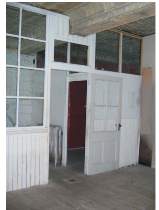
Figure 39: 284 William Avenue: Interior. (Sosa Fontaine, 2010).
