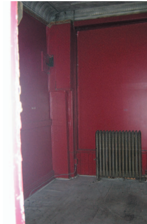
Figure 41: 284 William Avenue: Interior. (Sosa Fontaine, 2010).
