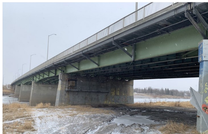
Fig 3.1. The South Perimeter Bridge
