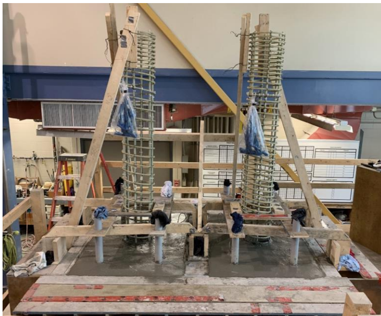
(a) Casting footings of the GFRP-RC columns G6 and G7
