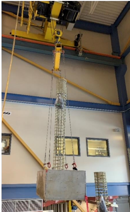
(a) Moving hardened footing
