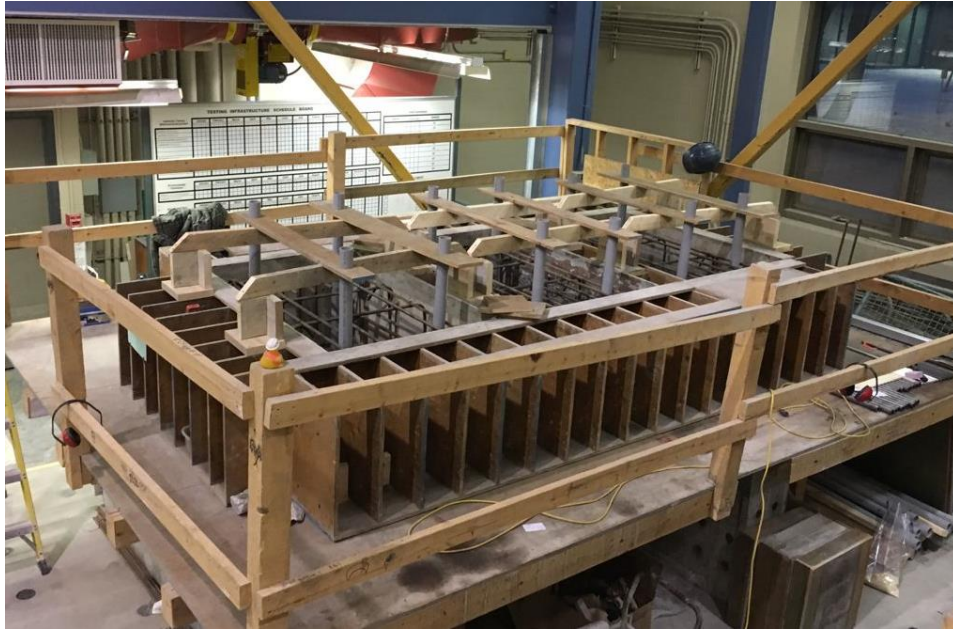
(b) Steel-RC cages and formwork of the footings in place
