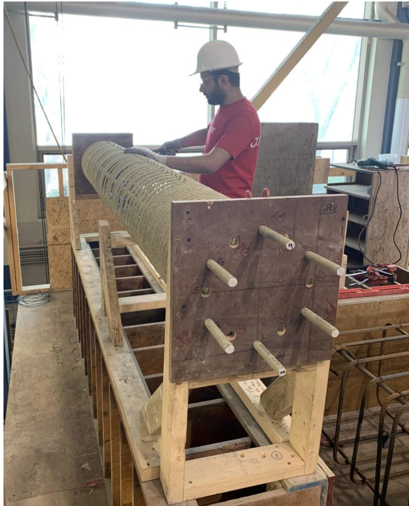
(a) Fabricating the GFRP-RC reinforcement cages
