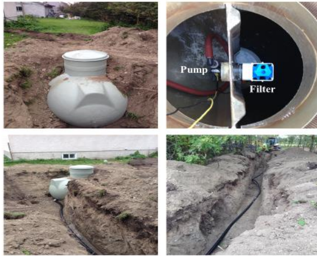
Figure 2.2 Septic tank installation
