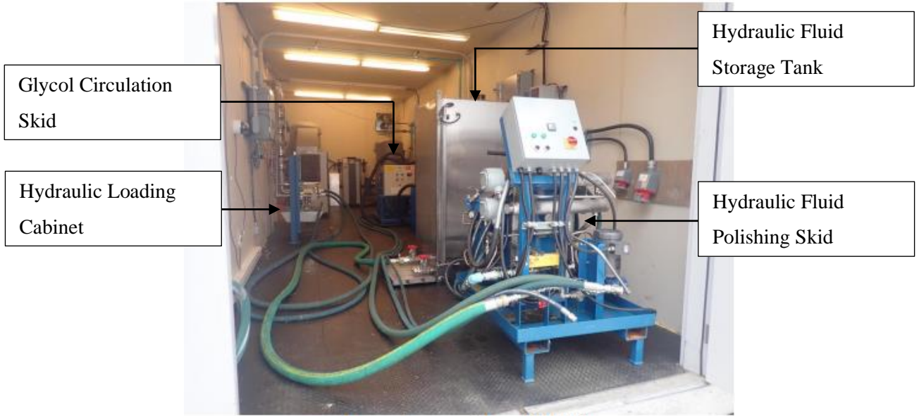
Figure 2: Current hydraulic loading room [2]
