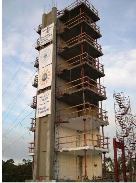
Figure 4-20: The building test structure [89].
