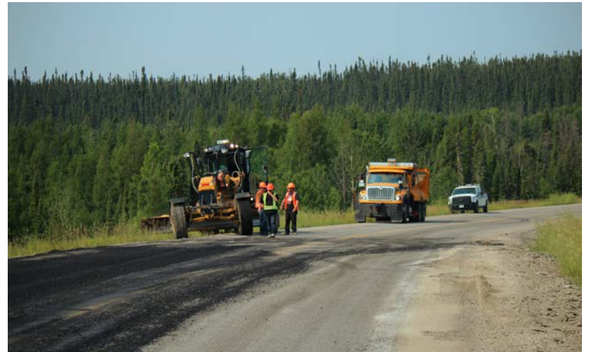
Figure 1-42: PR 391: grading.
