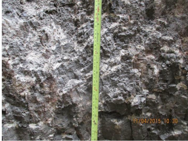
Figure 3.14 Silt pockets observed within fissured clay in a CBBD2 test pit
