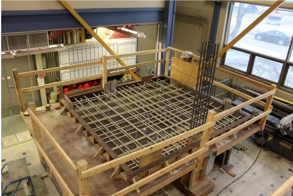
Figure 3.19: Specimen 2 (GFRP-RC with reinforcement ratio of 0.7%) before casting
