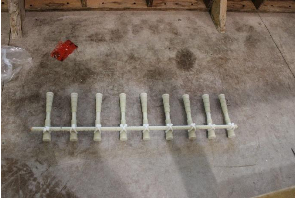
a) Shear studs' rail assembled
