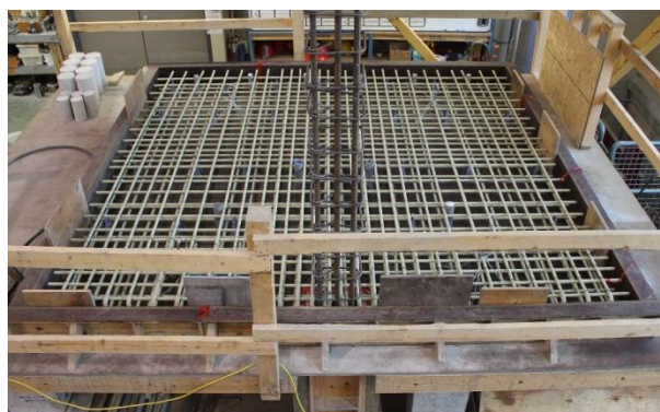
c) Connection before casting
