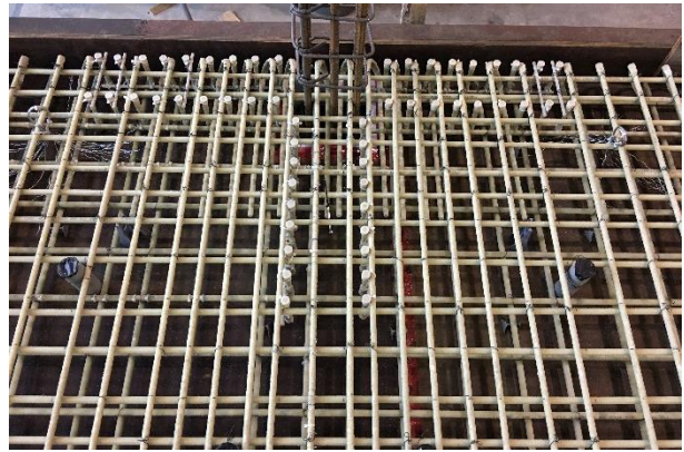
d) All reinforcement assembled
