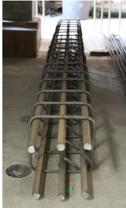
Figure 3.17: Column steel reinforcement cage
