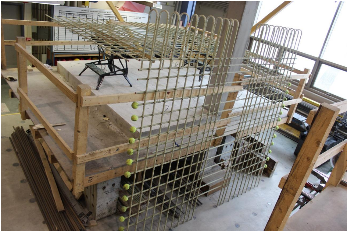
Figure 3.16: Assembled GFRP reinforcement assemblies
