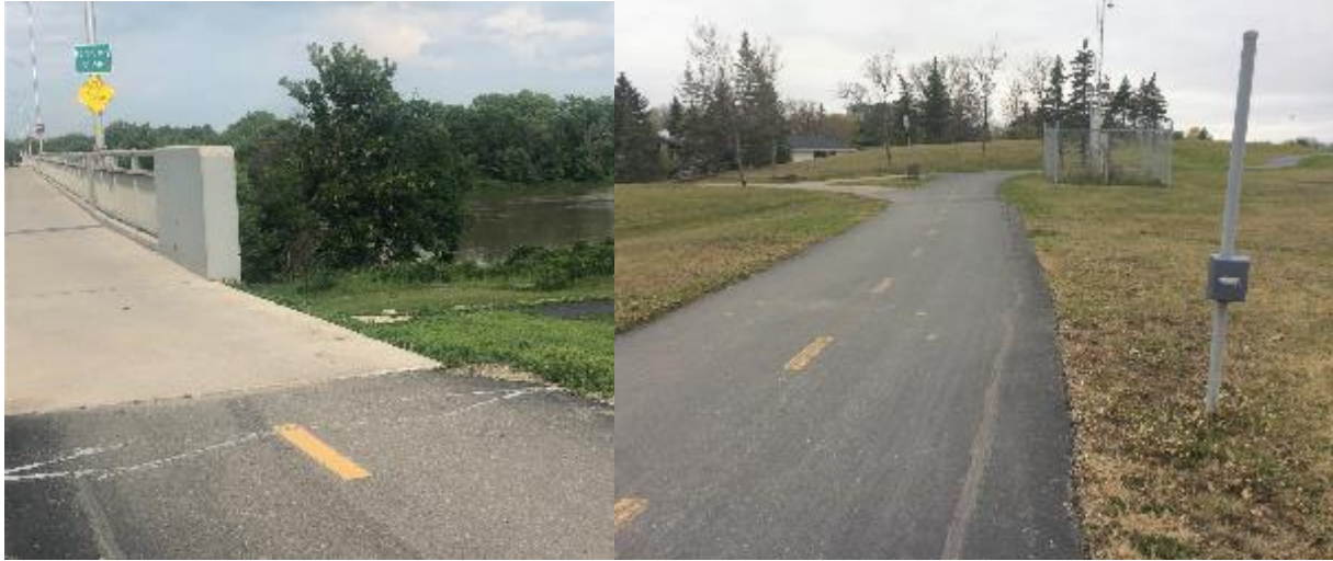
Figure 4.19: Bishop Grandin site ground view level (Left: inductive loop, Right: passive infrared sensor)
