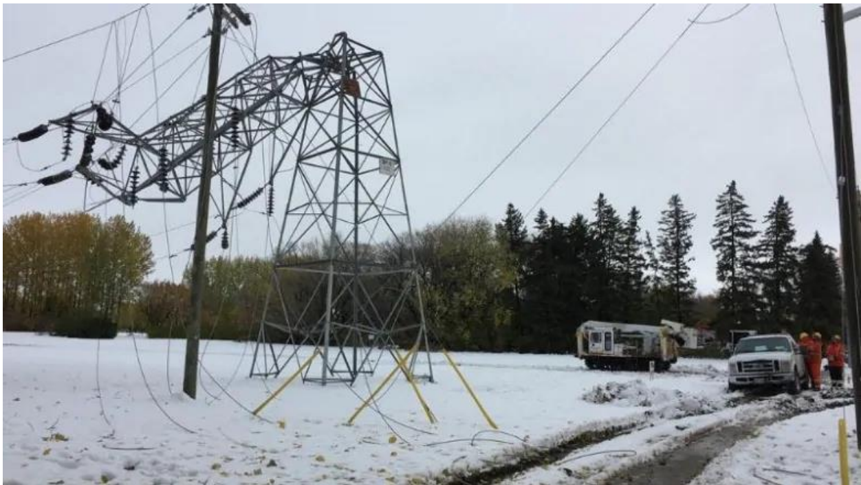
Figure 1.2: Collapsed Hydro tower as a result of a wet snowstorm on October 11, 2019. Photo by Manitoba Hydro, used with permission. Retrieved from: https://www.cbc.ca/news/canada/manitoba/manitoba-hydro-snowstorm-powerless-customers-residual-effects-1.5335157
