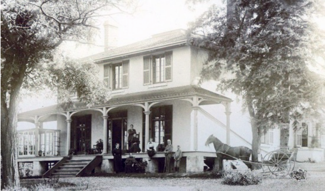
Figure 3.3: 'Ainslie Hill', the Anderson Family Home in Sutton, Ontario 53
