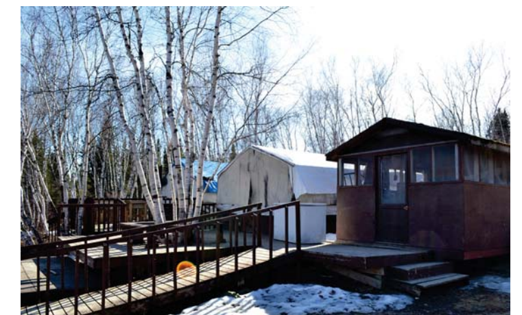
Exterior of group buildings for maintenance and eating
