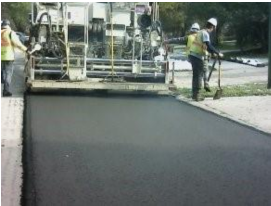
a) Site image during paving
