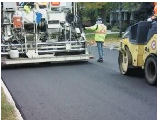
a) Site image during paving
