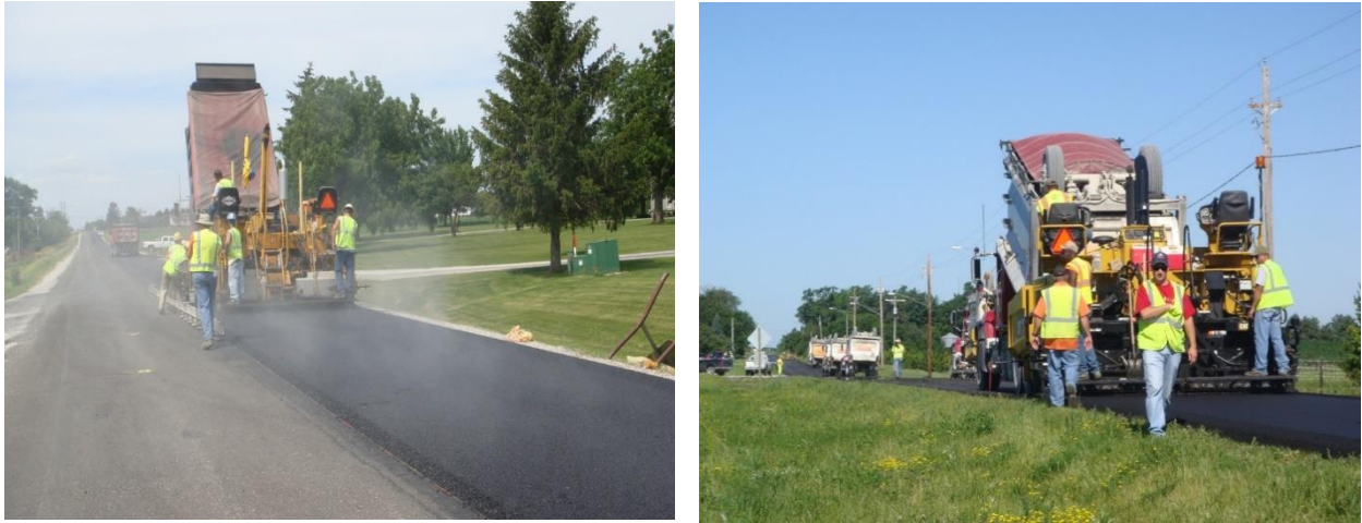
Figure 2.3 Paving using HMA technology (left) and WMA (right) (City of Winnipeg)
