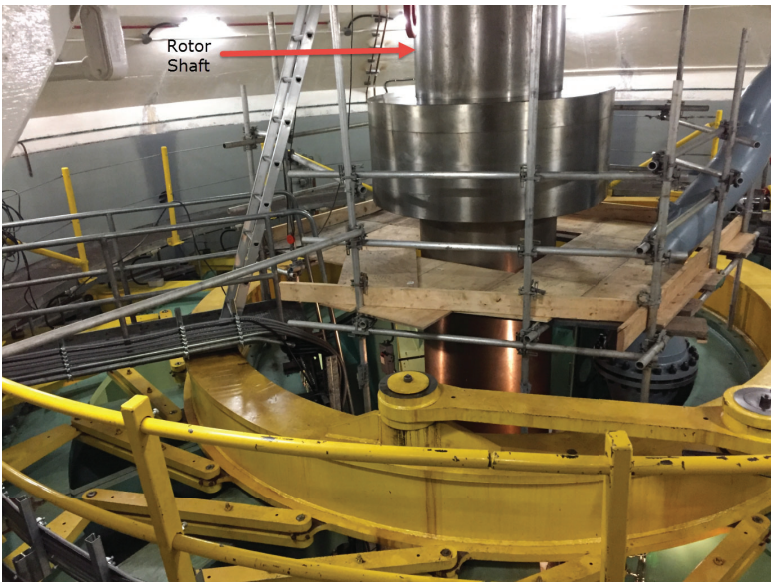
Fig. 1.1: Turbine pit of a hydrogenerator.
