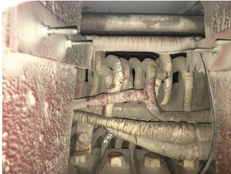
Fig. 6.6: View inside window behind slot 329 for measurement of A-phase PD.
