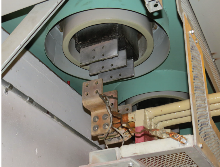
Fig. 1.5: Stator terminals (bottom) and isolated phase bus terminals (top). They are connected in-service.
