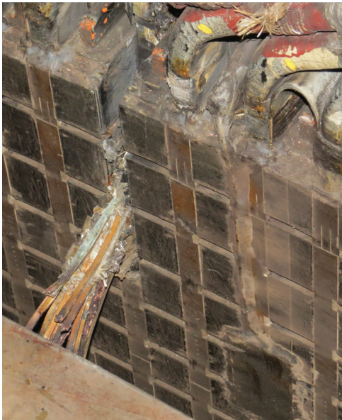
Fig. 1.13: Front view of failed coil that experienced a turn to turn fault.
