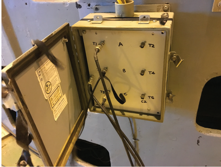
Fig. 6.1: Panel used for online PD measurements on Great Falls Unit 1. The triax cables from coupling capacitors enter at the top of the panel.
