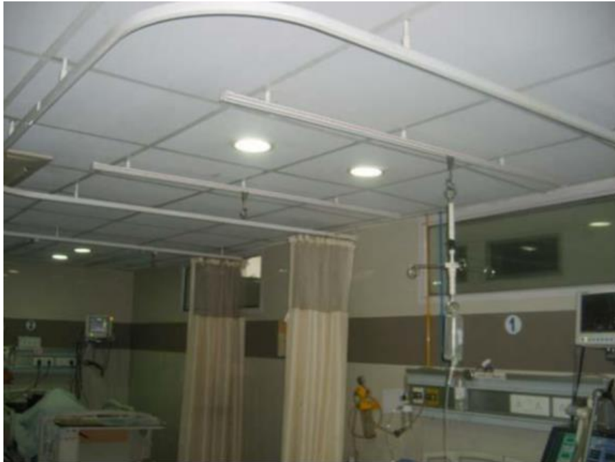
Figure 1: Exposed ceiling mounted tracks within an ED
