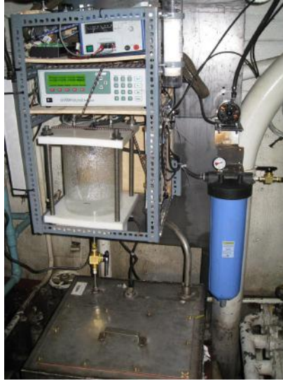
Figure 3: The on-track p\text{CO}_2 system located in the engine room of the Amundsen. The equilibration chamber is the clear cylinder (left bottom) and the gas analyzer is the box with the digital display.
