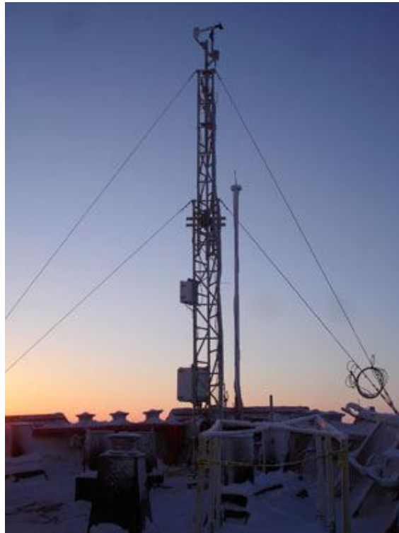
Fig.1. Meteorological tower installed at the front deck.
