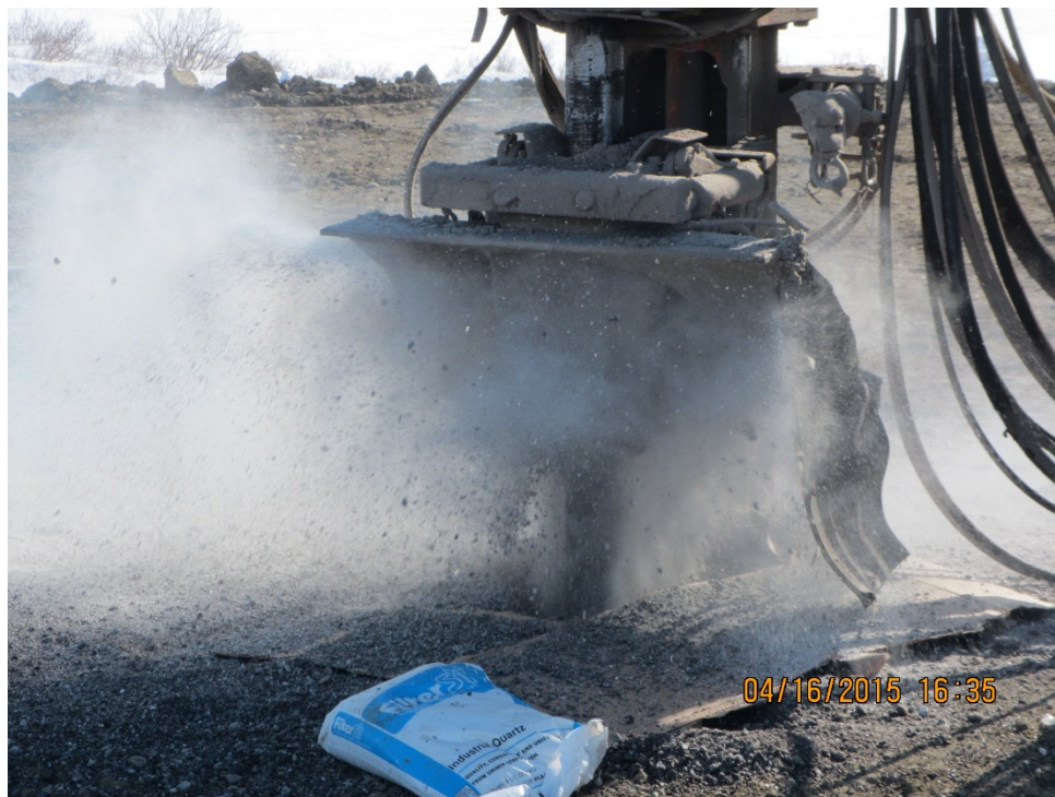
Photo 12: Materials jettisoned to surface by forced air during drilling with DTH rig
