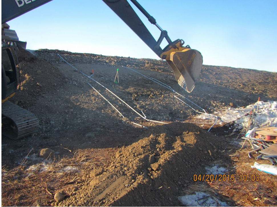
Photo 21: Protective conduits for instrumentation being covered with protective fill layer
