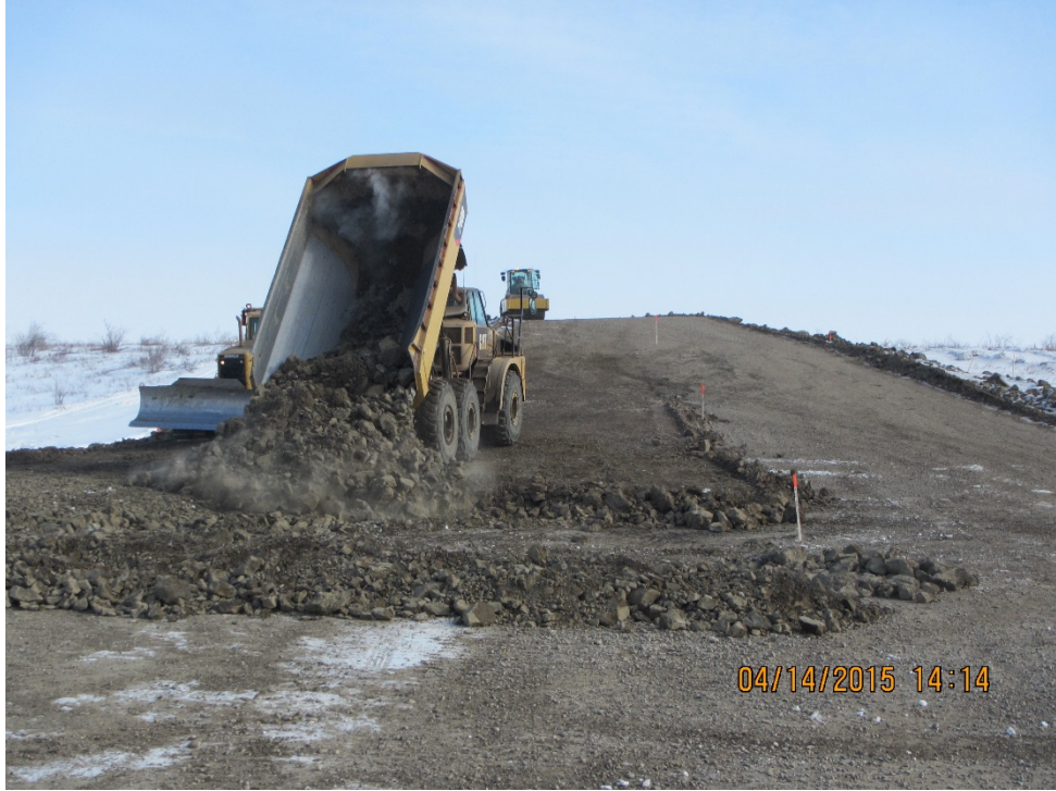
Photo 7: End-dumping of loose lifts of frozen granular fill
