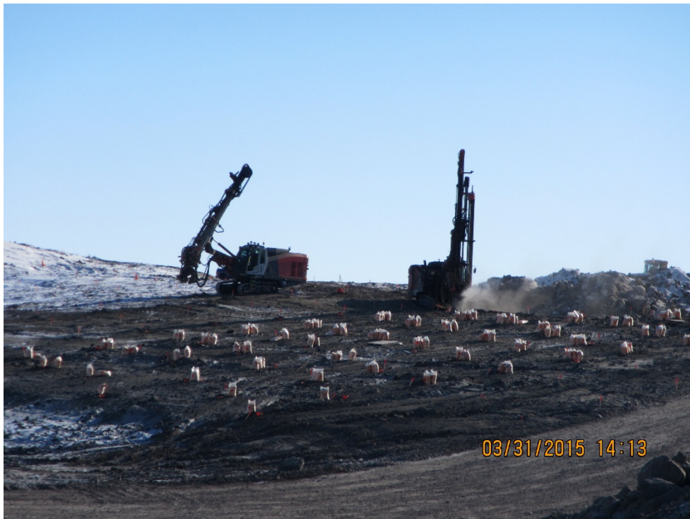
Photo 2: Drilling of blast holes in frozen granular fill at Borrow Source #174
