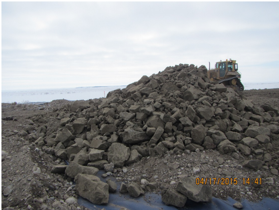
Photo 16: Typical type Nbe (Non-visible ice, well-bonded, excess ice) and Nbn (Non-visible ice, well-bonded, no excess ice), as delivered to site
