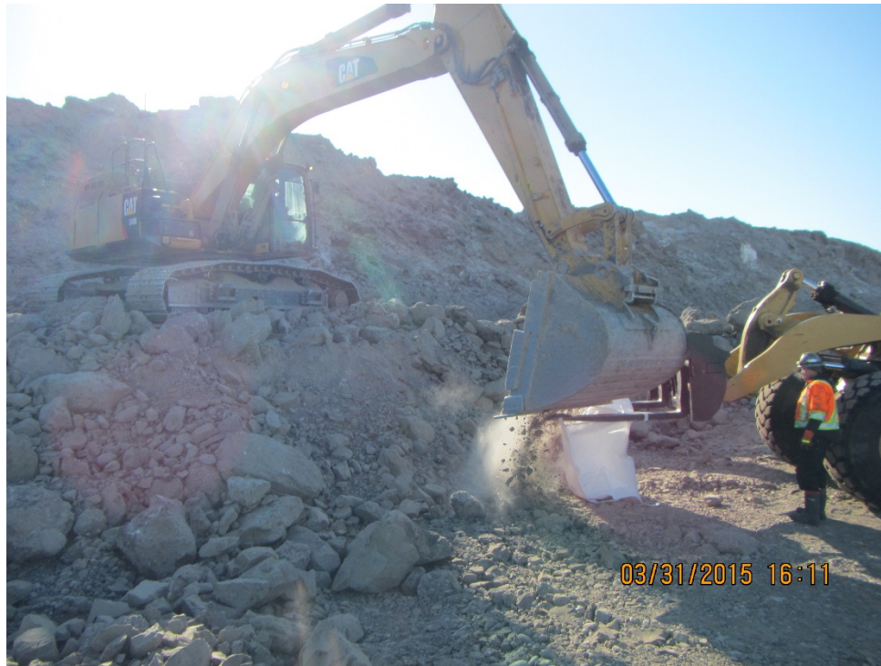
Photo 3: Collection of bulk frozen granular fill sample at Borrow Source # 174
