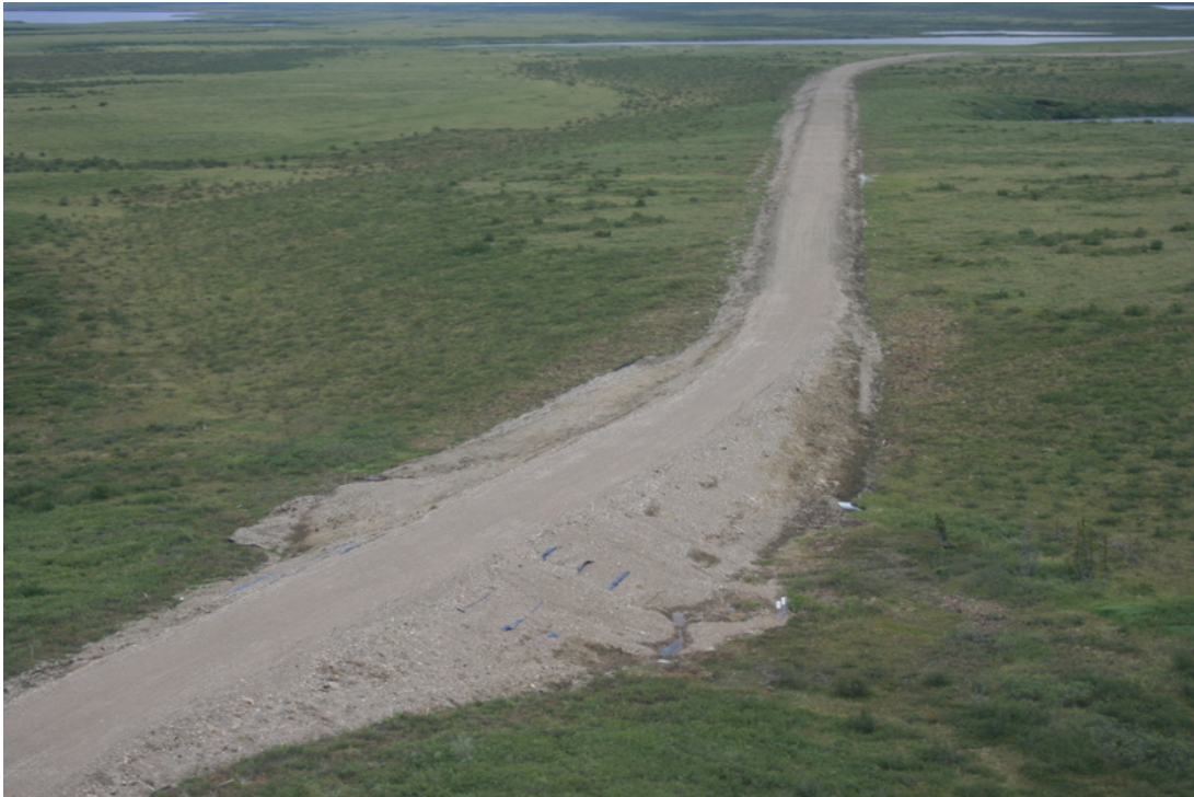
Photo 24: Overall view of test embankment looking southeast 2015/07/03, (photograph courtesy of Lukas Arenson)
