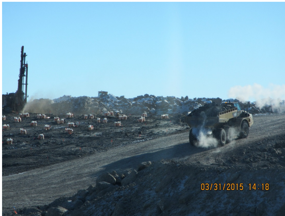
Photo 4: Hauling of frozen granular fill with rock truck from borrow source
