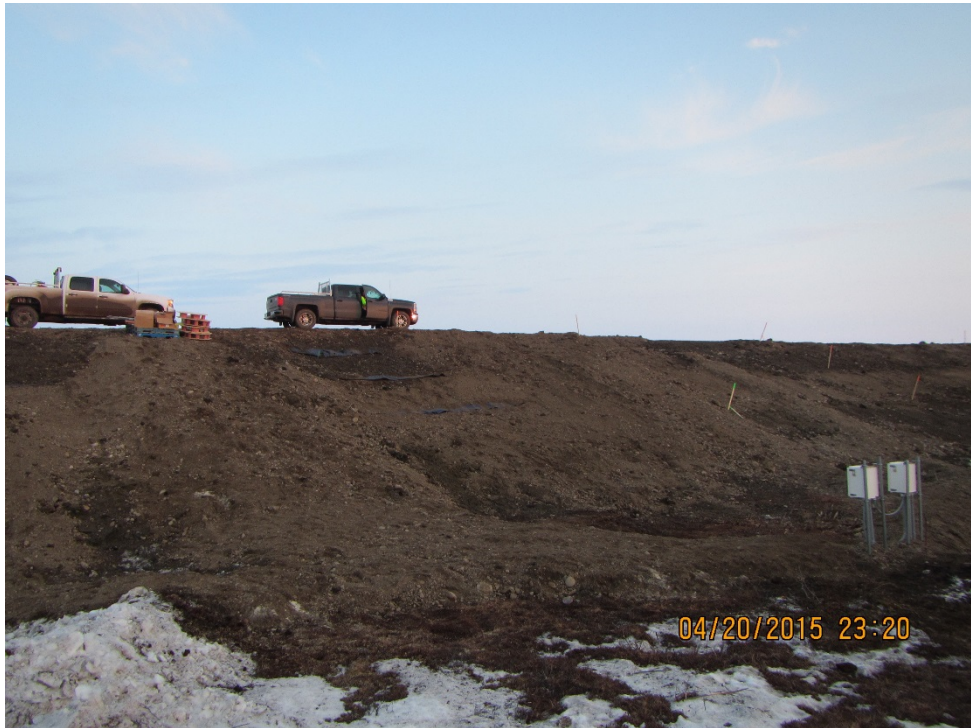
Photo 22: Completed test embankment, see instrument data acquisition boxes in right foreground
