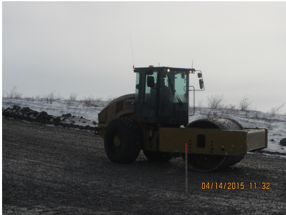
Photo 9: Compaction of frozen granular fill with vibratory roller
