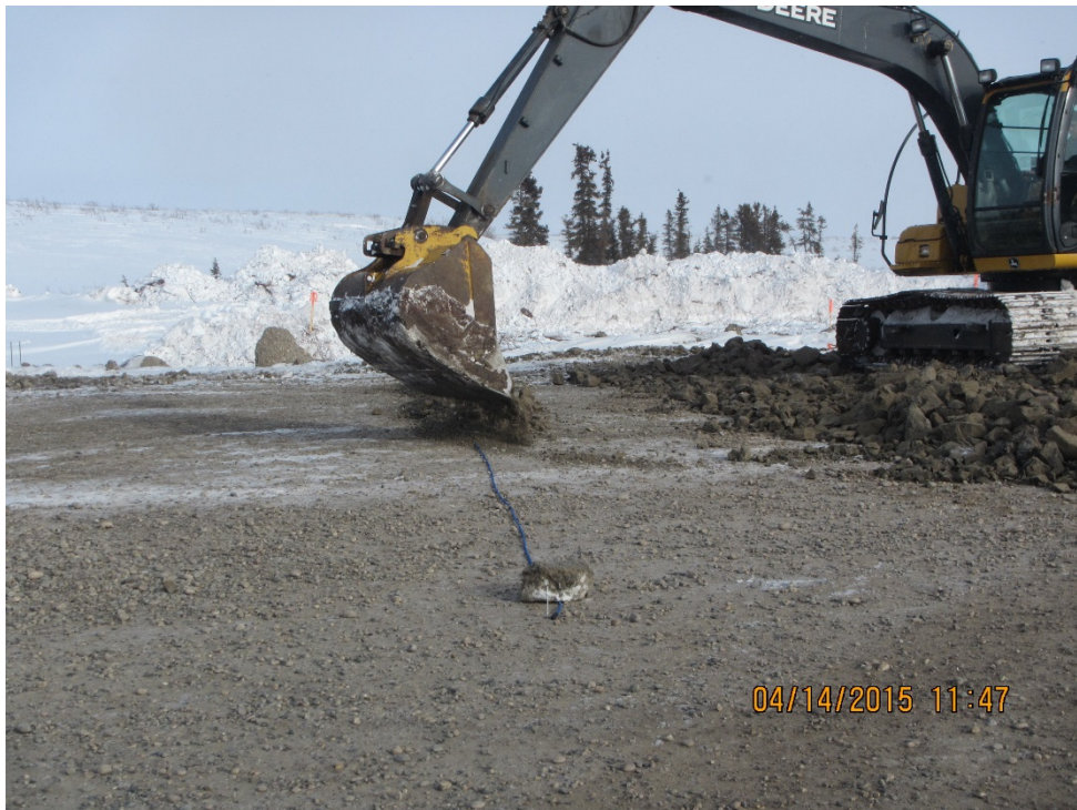
Photo 6: Placement of fill over thermistor string TS-C2
