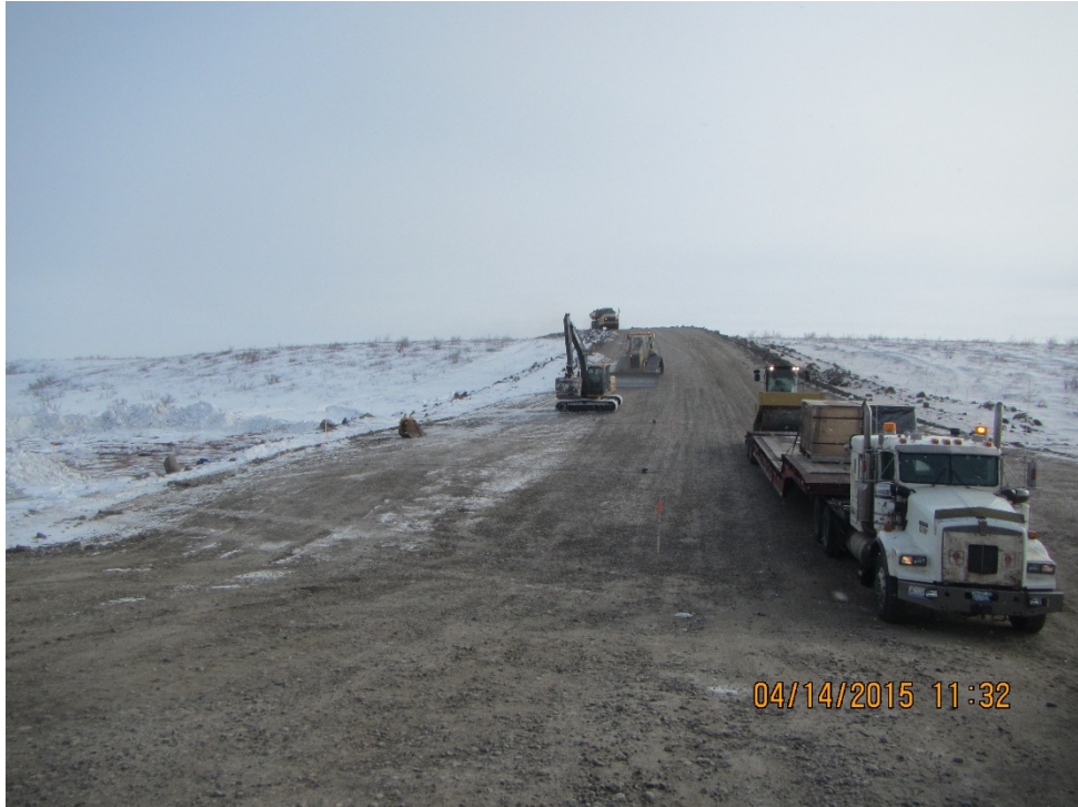
Photo 5: Test site prior to start of construction (looking north)
