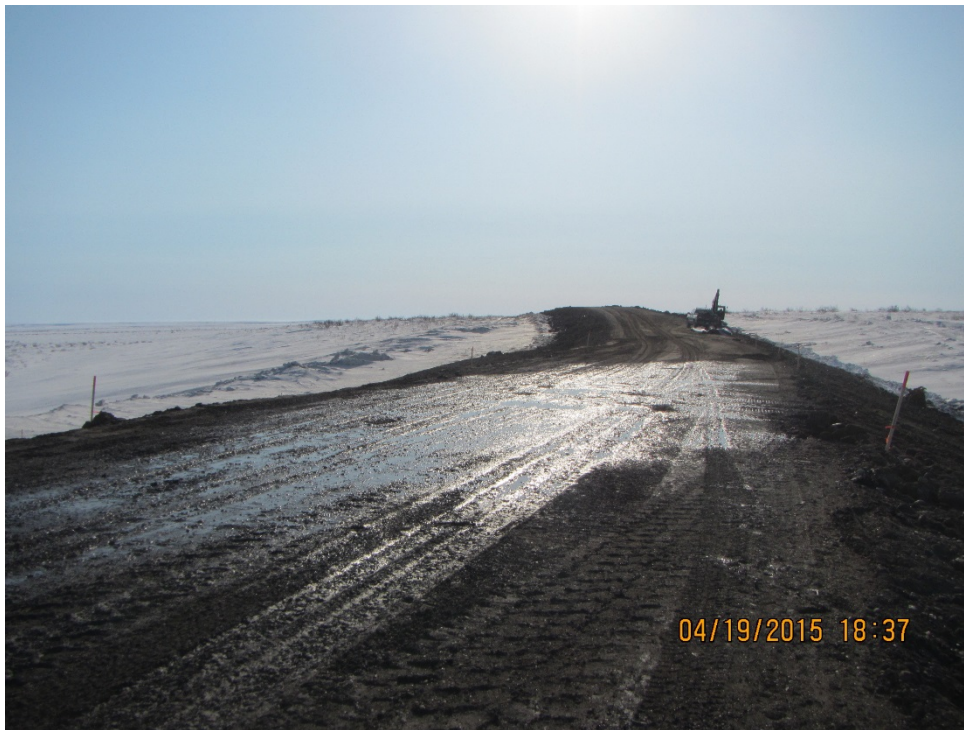
Photo 20: Thawing of exposed compacted fill surface on April 19
