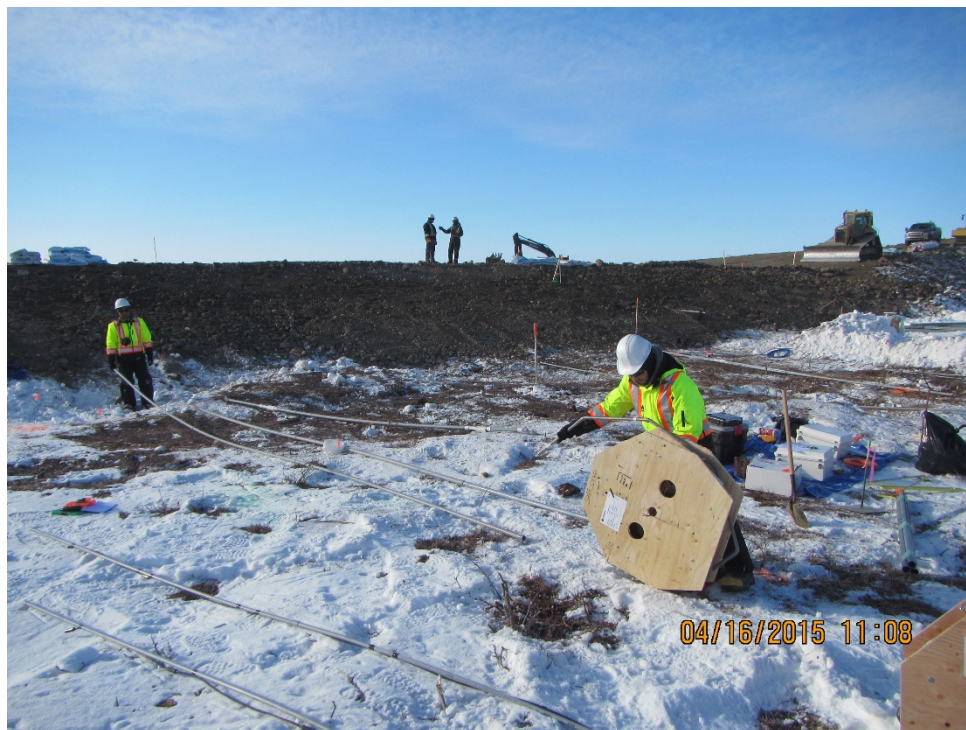
Photo 10: Preparation for SAA instrumentation installation. (embankment construction progress visible in background)
