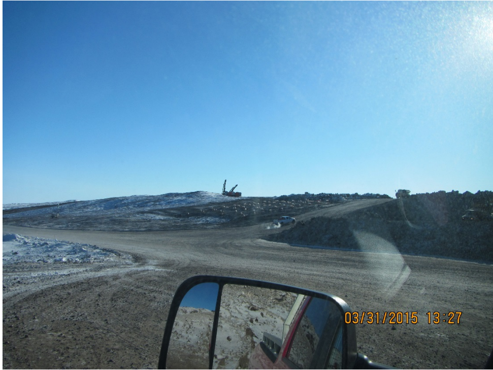
Photo 1: Preparation for blasting within an area of Borrow Source #174
