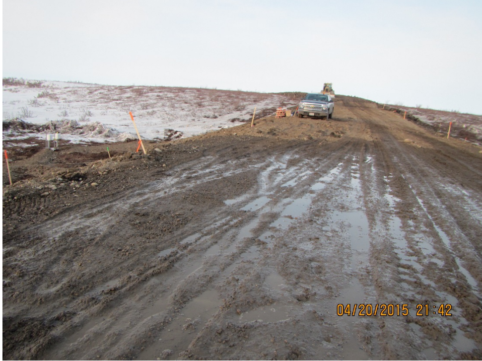
Photo 17: Supernatant water at soil surface following thawing at end of construction
