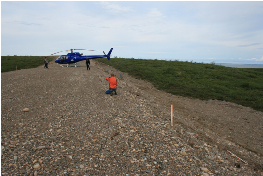
Photo 26: Longitudinal cracking along crest of test embankment 2015/07/03, (photograph courtesy of Lukas Arenson)
