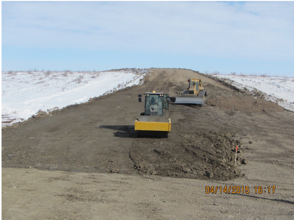
Photo 8: Breakdown and compaction of frozen granular fill with dozer and vibratory roller
