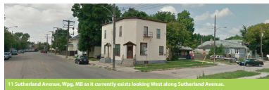
11 Sutherland Avenue, Wpg, MB as it currently exists looking West along Sutherland Avenue.
