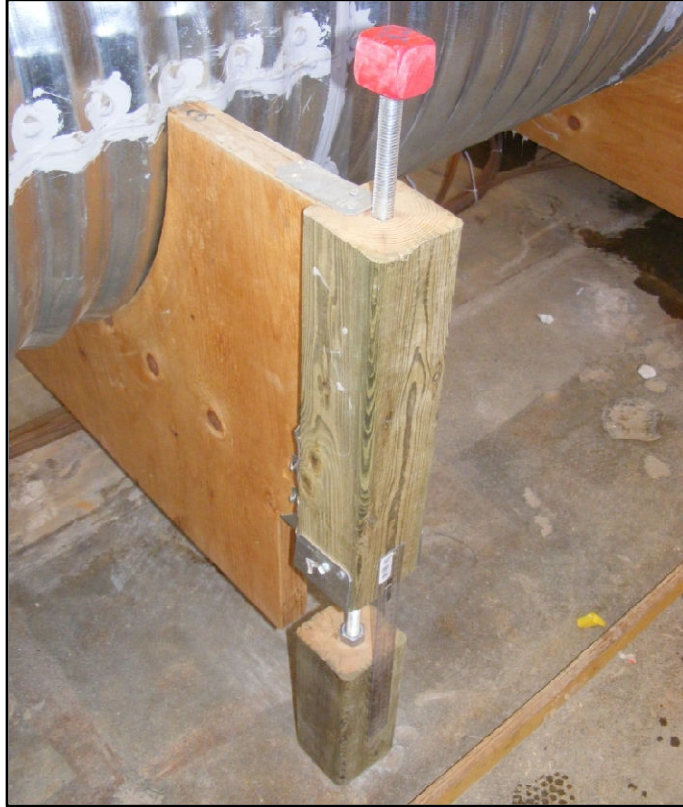
Figure 2.3 Culvert support post
