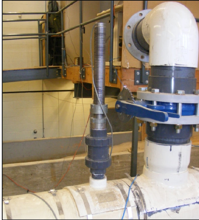
Figure 2.7 Magmeter installed on water supply line
