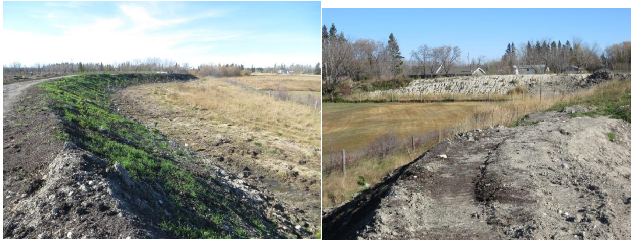
Figure 4. Views of the north side of the berm. This is where the off-farm drainage enters the property. The low vegetation cover (especially right) makes it easy to understand why erosion is currently a concern.
