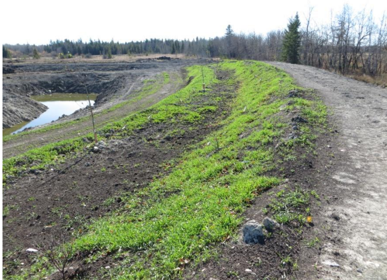
Figure 5. Interior of the northwest berm.
