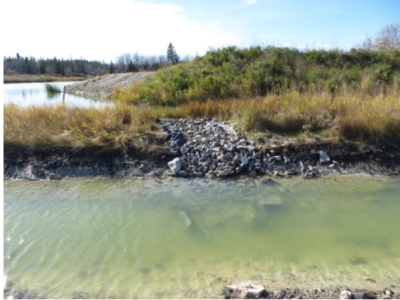
Figure 8. One of Bernie's suggestions was a protected overflow channel like this to keep the water level stable.
