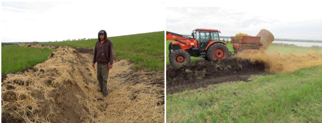
Figure 18. Takota giving a measure of scale in the top swale pictured left. On right, bale processor covering the swale with mulch (photo courtesy of Takota Coen).
