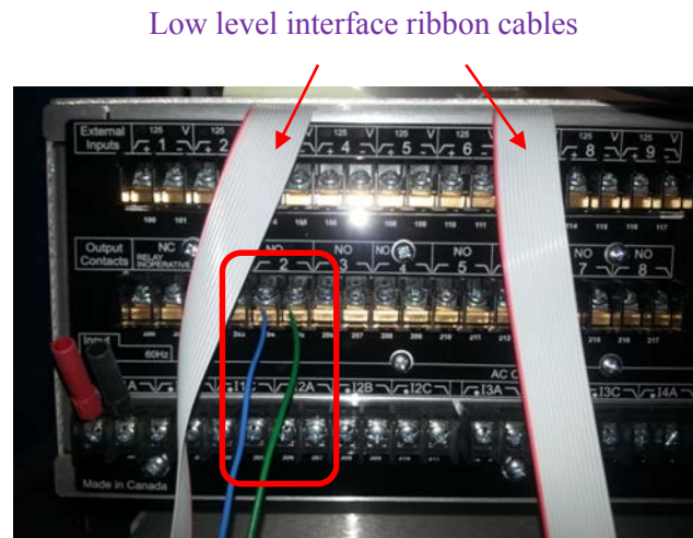
Figure 3-10: Hardwired connection of TPRO 4000 relay
