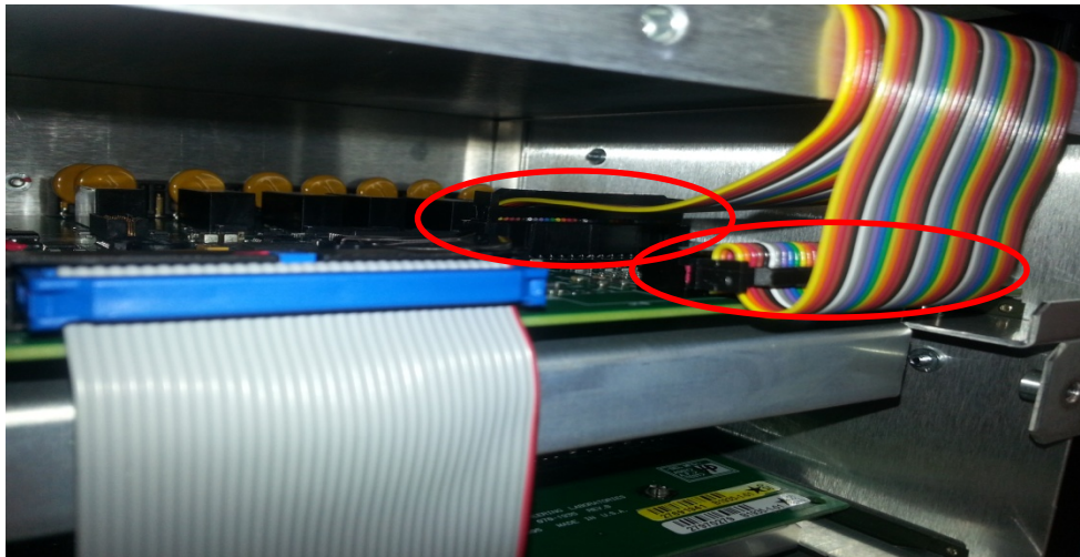
Figure 3-5: Low level interface of SEL 487E relay directly connected to RTDS with ribbon cables
