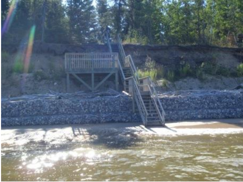
Modification: rock gabion retaining wall/sand beach Segment 38 photo B. MacDonald
