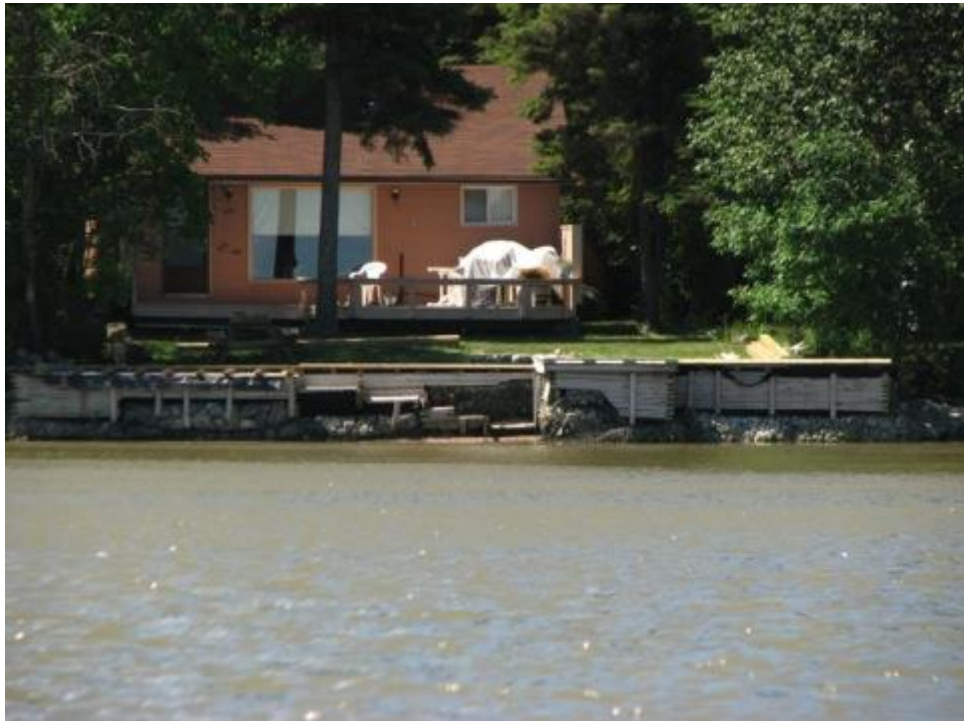
Modification –wood/rock retaining wall
