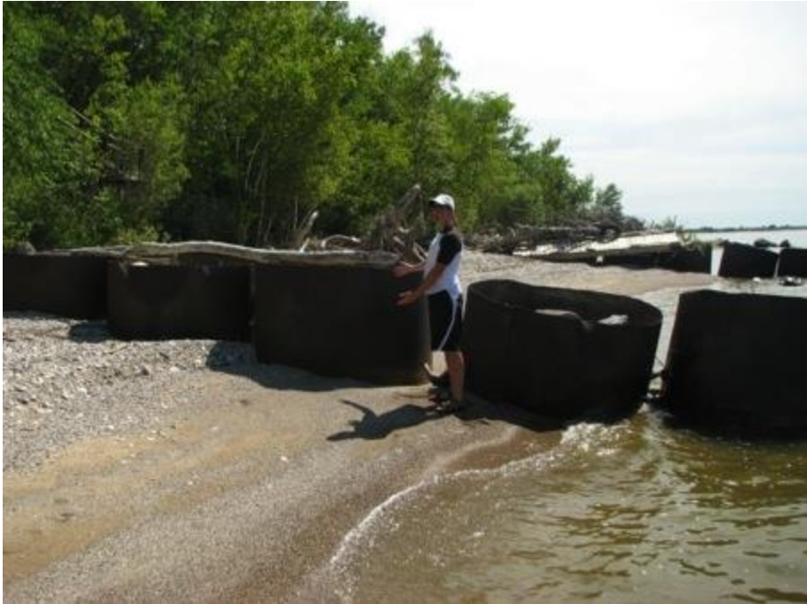
Modification: steel shoreline groyne Segment 30 photo P. Bloom
