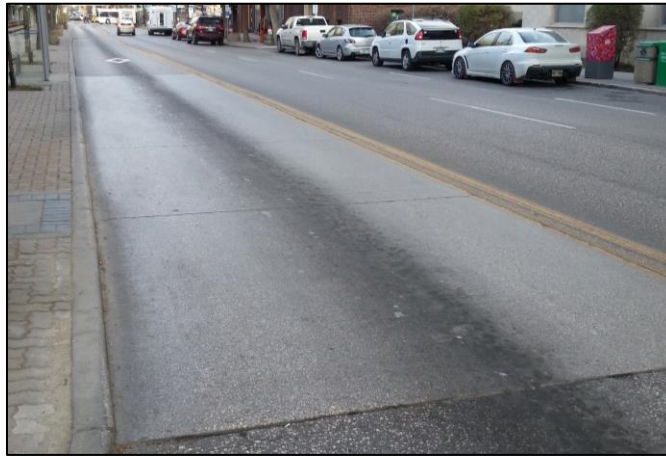
Figure 4: Concrete Pad at Bus Stop
