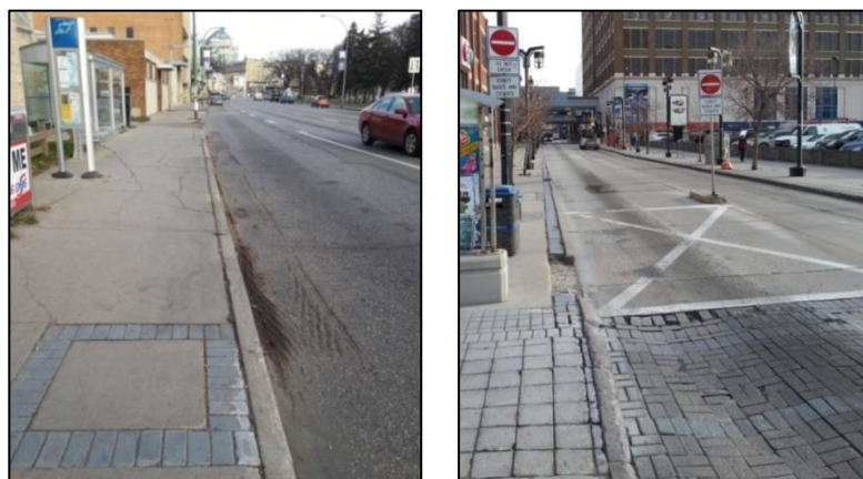
Figure 1: Examples of Transit Bus-Related Pavement Damage
