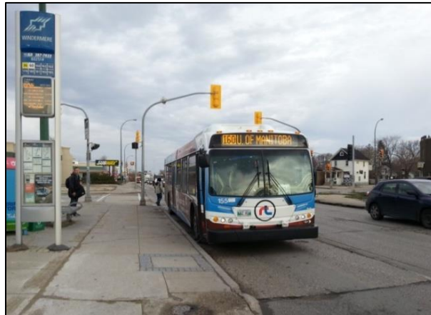
Figure 10: Portland Cement Concrete Pad at a Bus Stop on Pembina Highway
