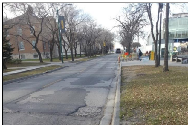
Figure 11: Asphalt Overlay on Dafoe Road
