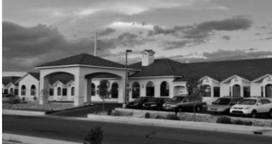
Figure 2.8.4.1 Exterior Façade, The Retreat
