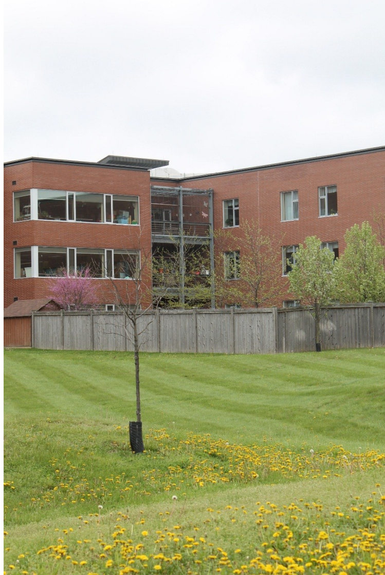
Figure 4.12.3 Exterior View, McCormick Home
