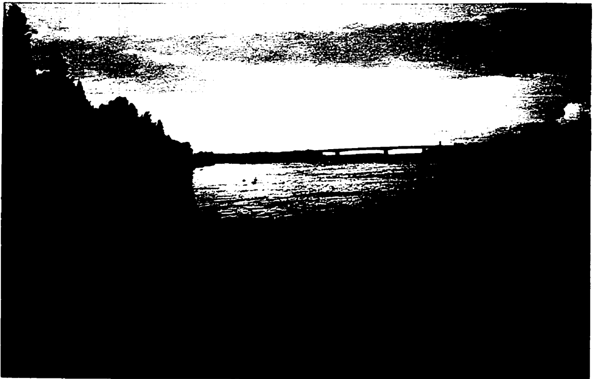
Plate 1 Grand Rapids Bridge. The bridge spans the Saskatchewan River and joins the two aboriginal communities.
