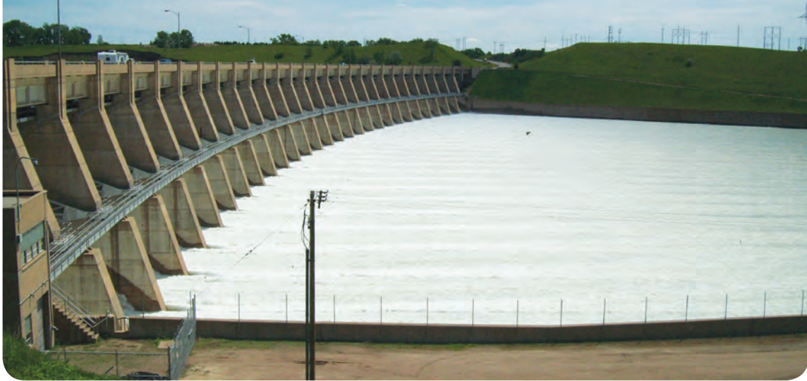
Spillway at Garrison Dam, June 19, 2011. Photograph by Stacey Gerhardt, USGS.
