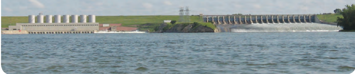
Powerhouse (left) and spillway (right) at Fort Randall Dam, June 9, 2011. Photograph by Joel Petersen, USGS.
