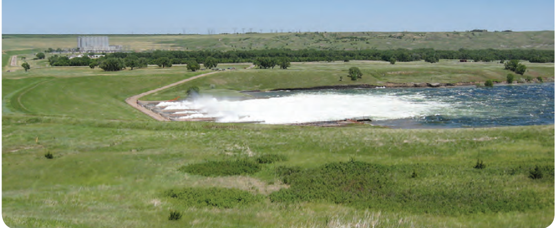
Oahe Dam (powerhouse in background), June 7, 2011. Photograph by Joel Petersen, USGS.
