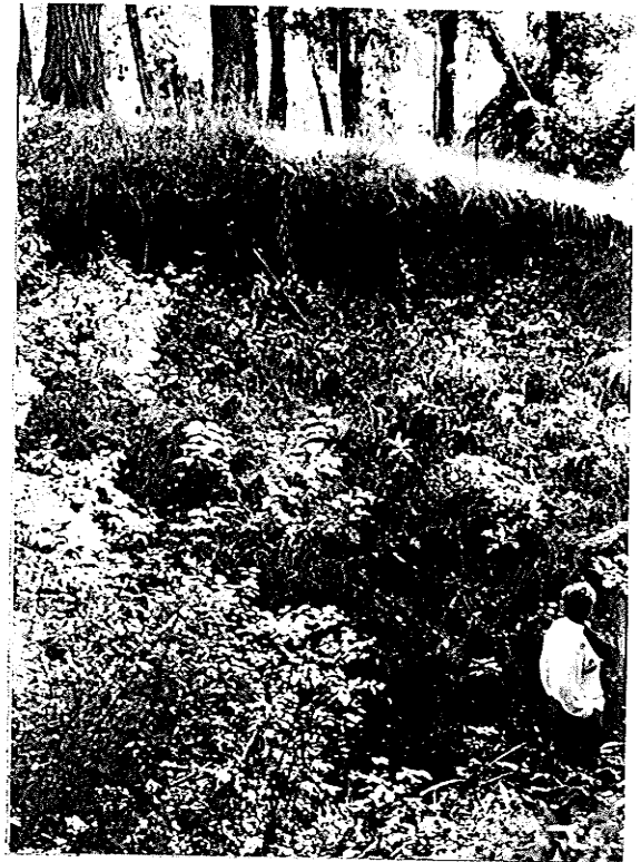
Photo P-13. Erosion south of South Bridge (Sept 25, 1993).
