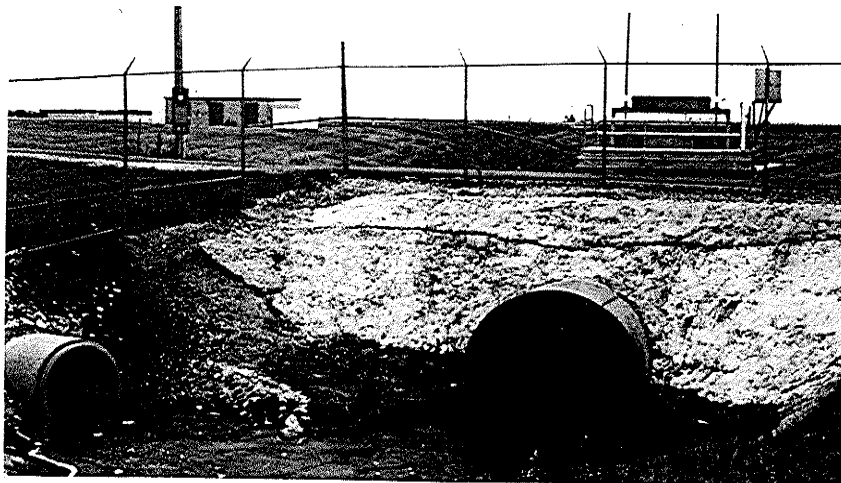
Photo P-8. The Pollution Control Structure at airport outlet (Nov 3, 1993).
