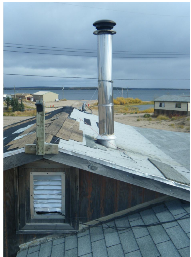
Figure 4: Roof repairs on one house in Tadoule Lake. Photo © Larcombe 2010
