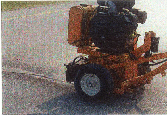
FIGURE 3.2: Routing of Crack to a 3:1 configuration
