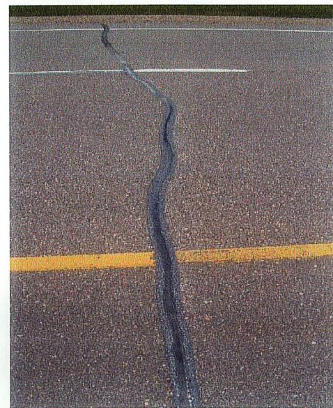
FIGURE 3.7: Final Sealed crack across the entire road surface
