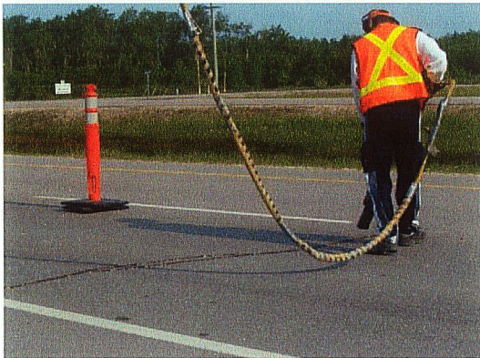
FIGURE 3.4: Heating of the crack using a hot-air lance
