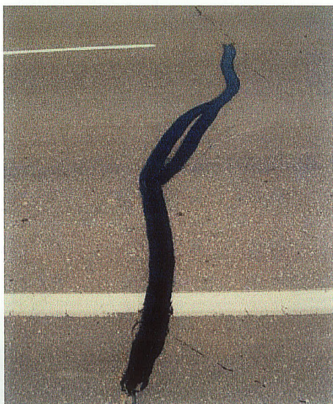
FIGURE 3.6: Final sealed crack
