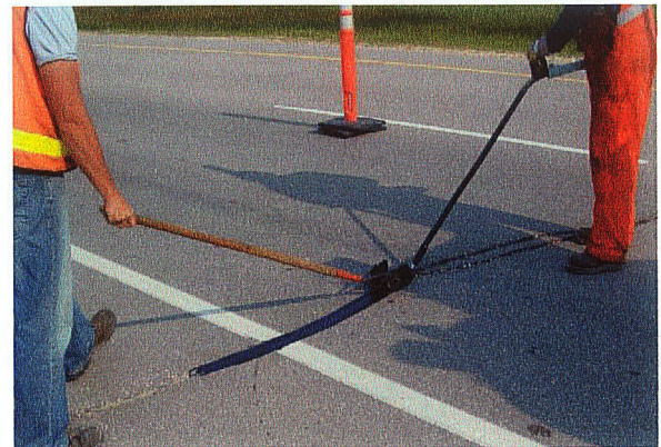
FIGURE 3.5: Sealant application using a wand and squeegee
