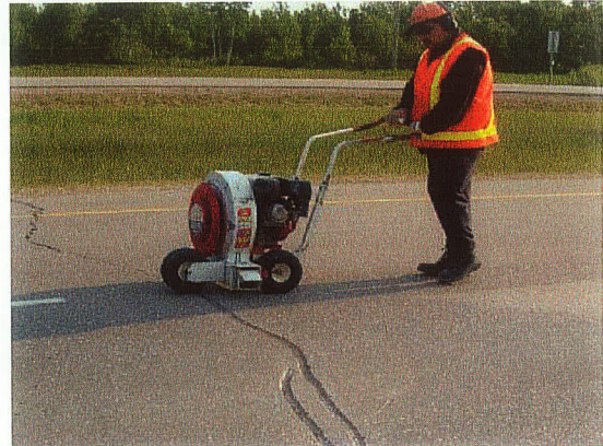
FIGURE 3.3: Cleaning of the crack using an air blower
