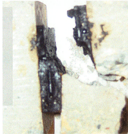
FIGURE 4.310B: Close up of failure within the sealant
