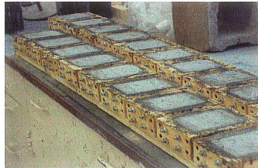
FIGURE 3.11: Concrete blocks after pouring
