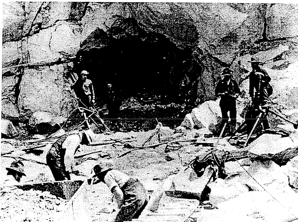
Figure 2.10. Construction of Buntzen Tunnel, circa 1902
