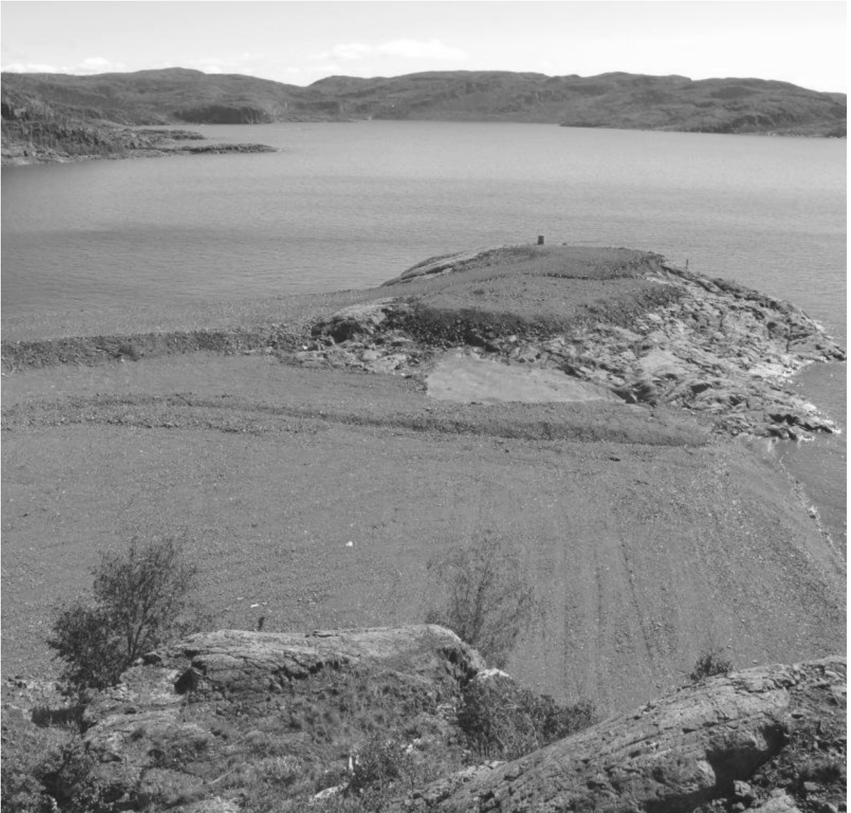
Figure 61: Port Radium, post-remediation - the site is covered with waste-rock Credit: Dawn Curtis / AANDC
