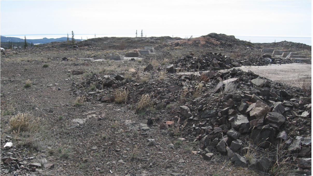
Figure 49: remnant concrete foundations from former site operations, Port Radium, 2007 Credit: Louis Covello
