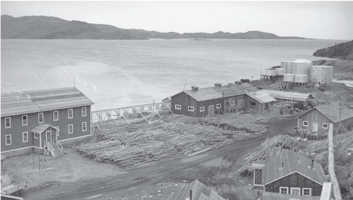
Figure 41: Eldorado pitchblende mining camp at Port Radium, Echo Bay, Great Bear Lake, 1939 ©Finnie/NWTArchives/N-1979-063-0080
