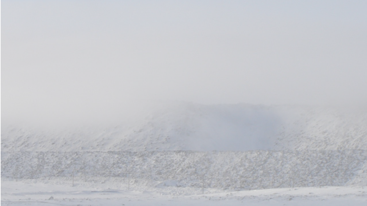
Figure 22: waste-rock pile at Diavik Diamond Mine, NWT - the human made relief creates a unique microclimate on the otherwise flat tundra (2006)
