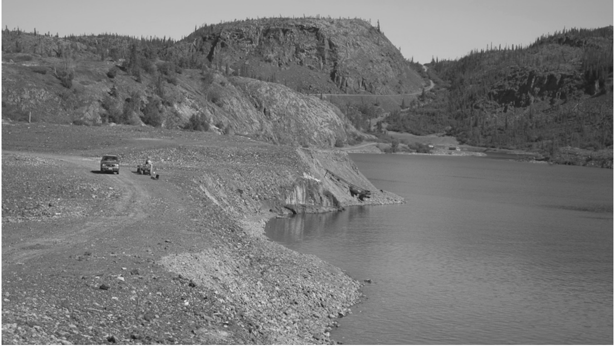
Figure 59: remediation activities 2007-2009 Credit: Colin MacDonald
