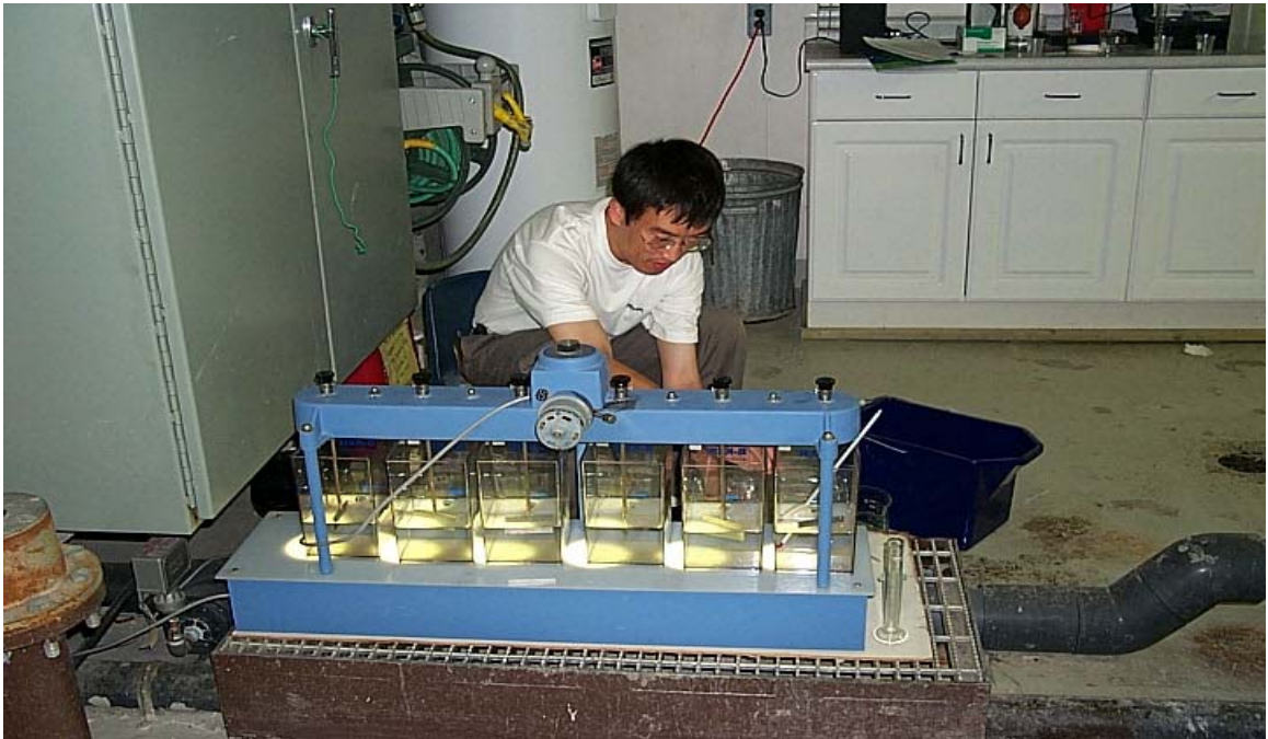
Figure E-2 Coagulation jar tests at the Split Lake WTP
